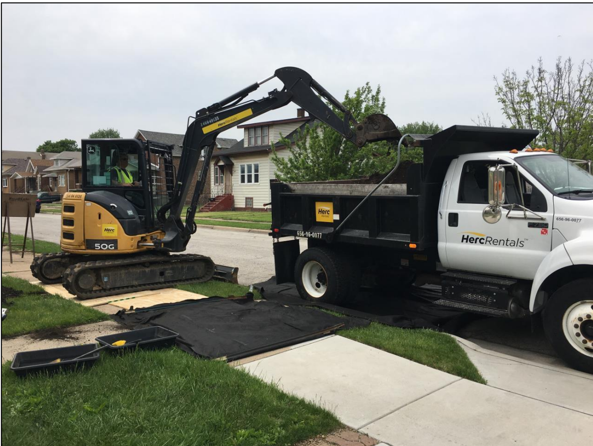
This is what typical soil excavation work looked like in yards near Federated Metals. Grass, trees and vegetation were restored after the contaminated soil was removed.
