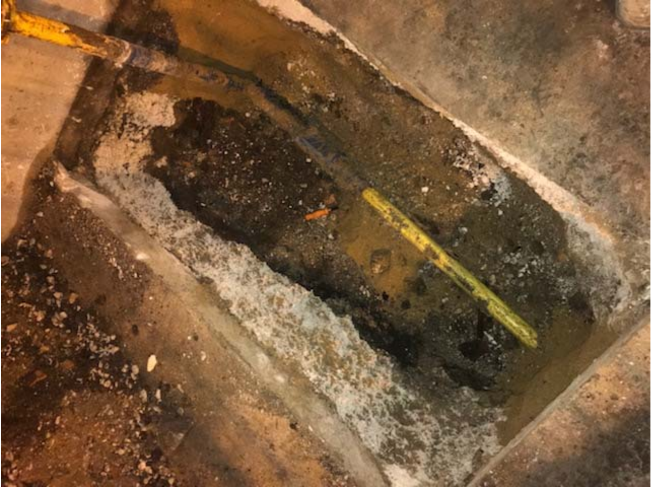
Photograph of 3 X 5 foot excavation prior to service line replacement.
