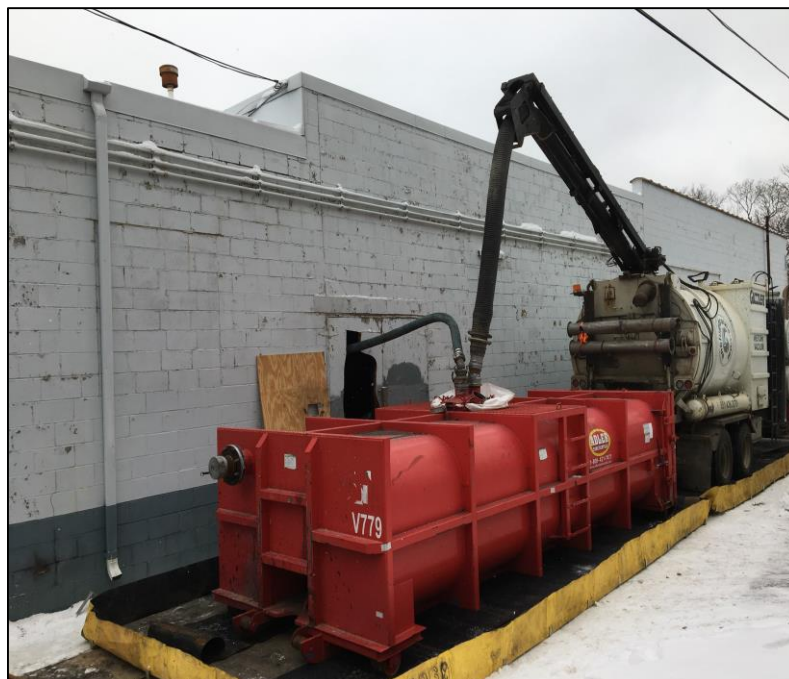
EPA used this equipment to remove acid sludge from vats at the Plating Inc. cleanup site in St. Paul, Minn.
