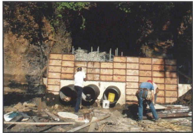
Figure 18. A hydraulic wet seal was constructed with a gravel bulkhead for water and subsidence control (Douglas Abandoned Mine Land Reclamation Project).
