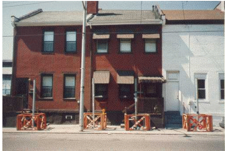
Figure 22. Vent stacks outside of residential structures.
