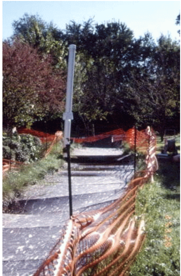
Figure 19. Water well vent.
