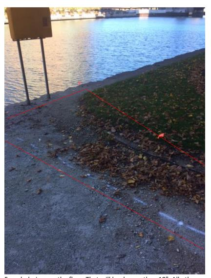
French drain near the flags. That will be deeper than 18". All other areas are painted and will be under 18" of excavation.
