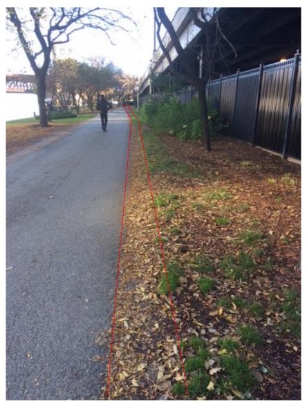
Along south side of path we are excavating under 6" and adding screenings and edging from Columbus bridge to lakeshore. Same as is on the north side
