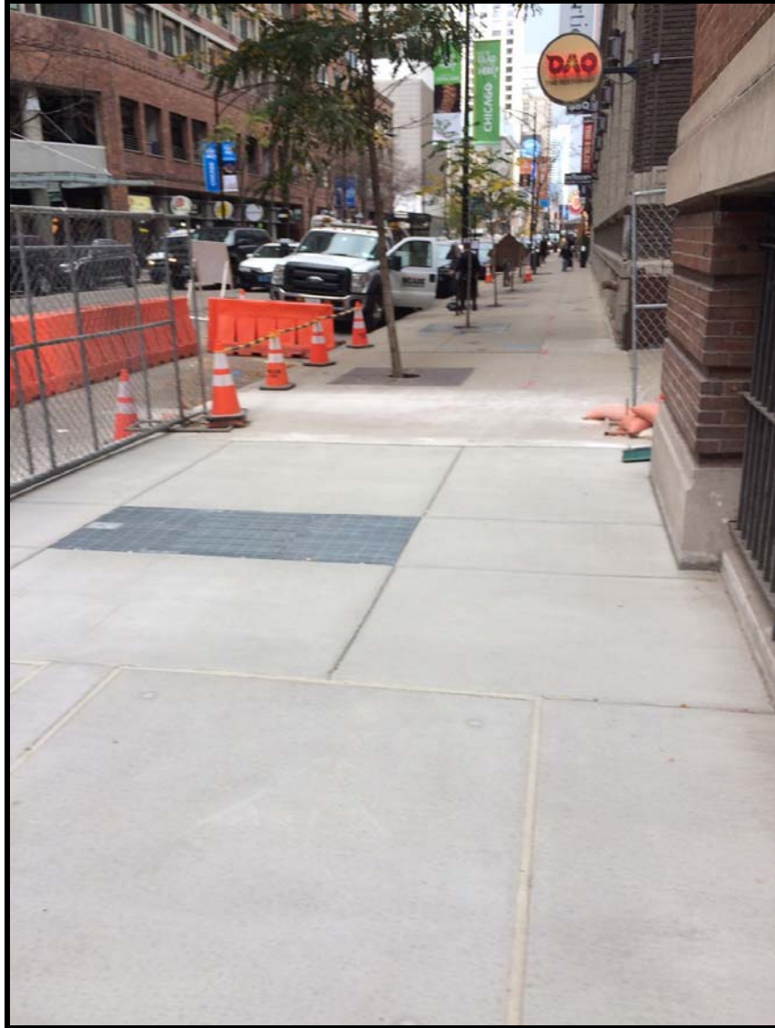
3) Photograph of completed sidewalk taken on 11/28/16 as barricades and fencing were being removed to reopen the sidewalk to pedestrian traffic.
