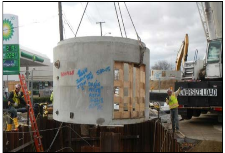
Installation of new vault at Bon Brae Street and Harper Avenue in November 2015
