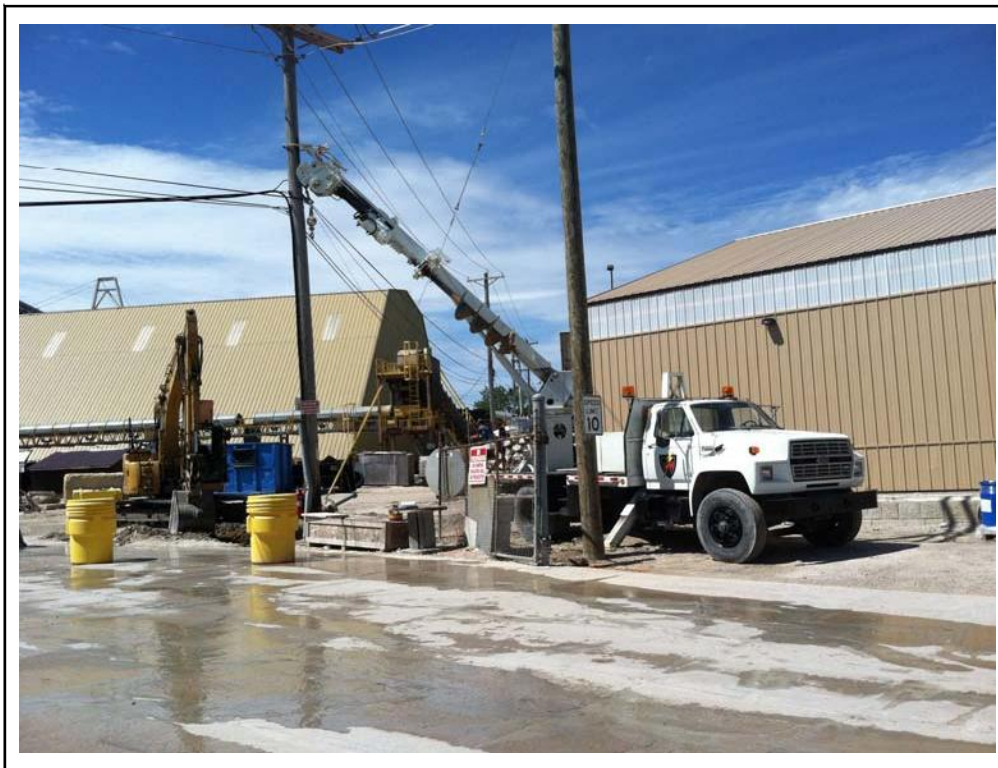
Photo No. 2: Power pole support during excavation.
