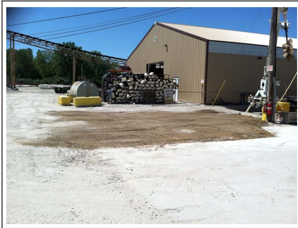
Photo No. 9: Finished excavation filled to grade.
