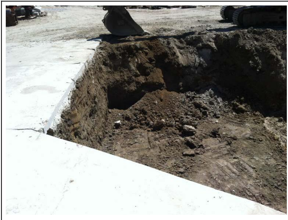
Photo No. 4: East side of excavation at concrete sawcut.
