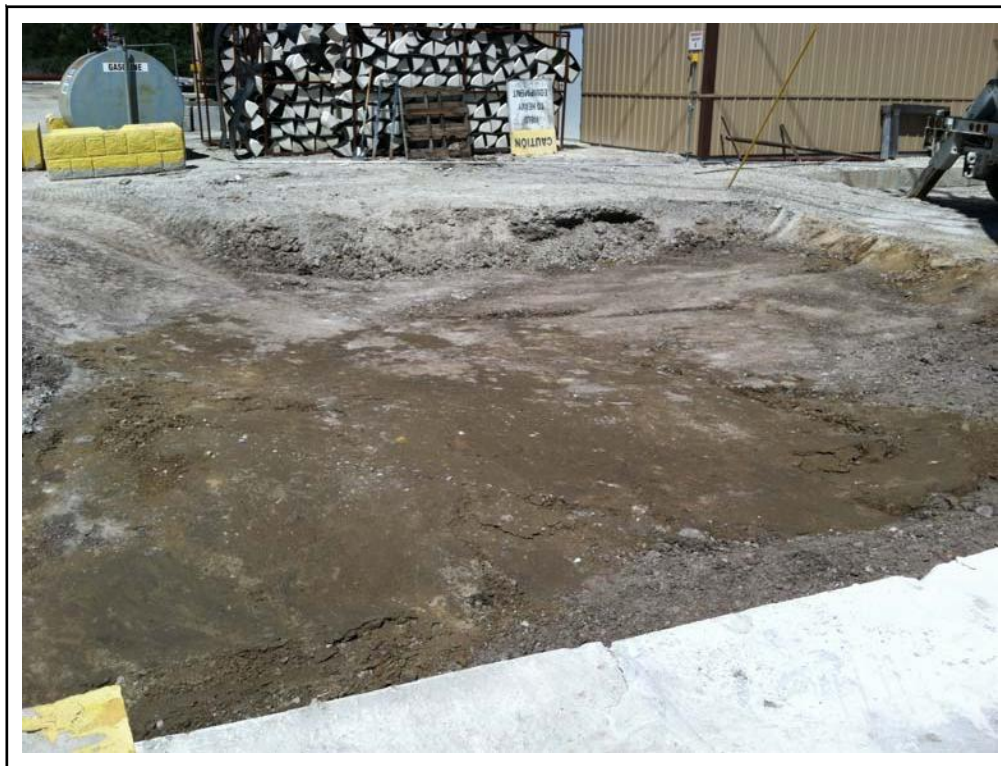
Photo No. 8: Top of clay cap.
