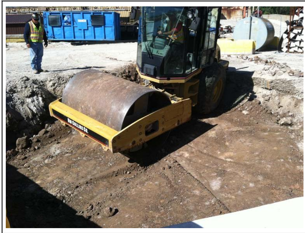
Photo No. 7: Compacting clay backfill with vibratory roller.
