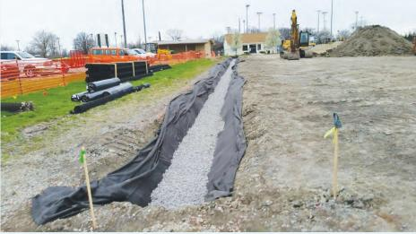
ture to the right show bioswales being installed. Bioswales will be located along three sides of the parking lot to catch more runoff from the parking lot. Bioswales are channels that have been designed to provide treatment and retention as they move stormwater from one swales slow, infiltrate, and filter stormwater flows. You may also see them designed with rocks or gravel. As linear features, vegetated swales are particularly suitable along streets and parking lots.
