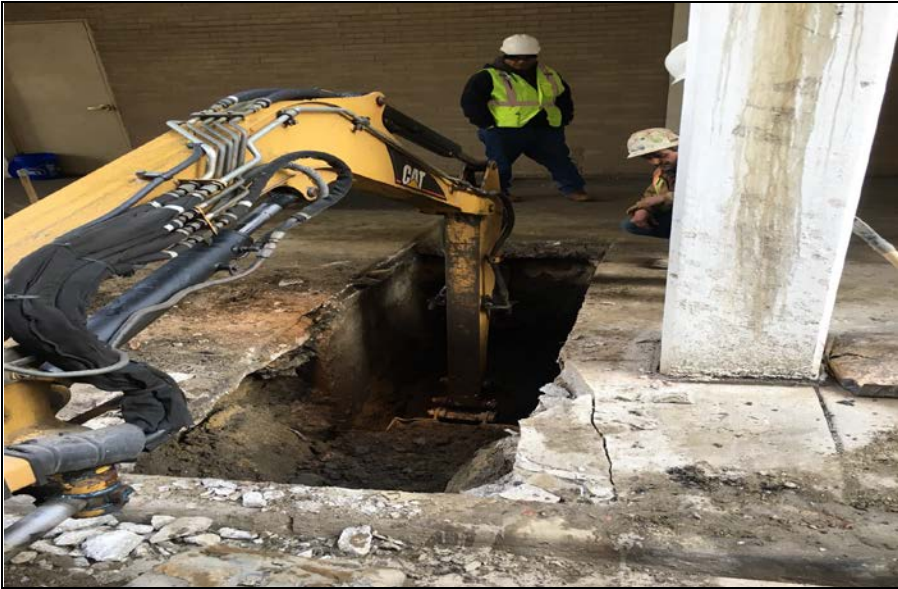
Photo 5: View facing north of excavating sidewalk for second break in sewer line
