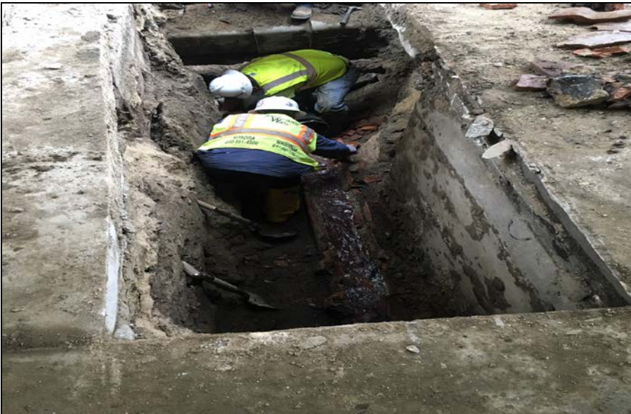
Photo 7: View facing south of removal of clay sewer line while active
