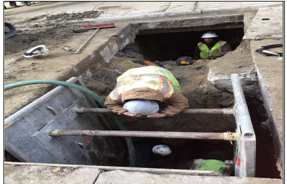
Photo 4: View facing north of pumping out excavation
