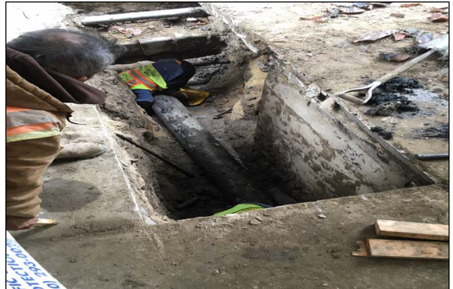
Photo 8: View facing south of installing new sewer line
