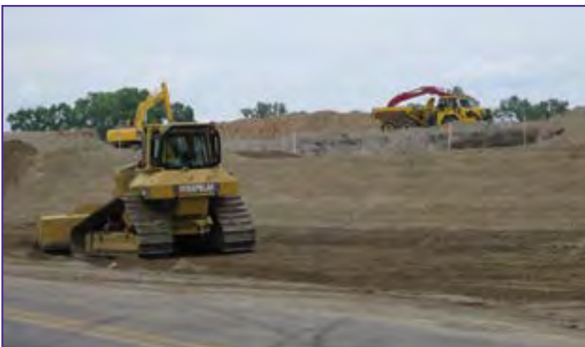
Grading the berm located along Blackjack Road
