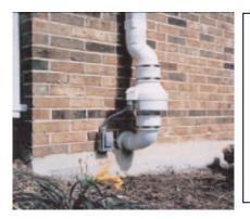
**Sub-slab mitigation system:** This system draws radon and other vapors out of the soil and vents them outside
