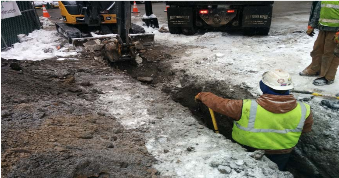
Photos - 419-20 E Ohio Street Service Installation
