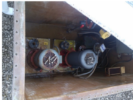
Pump motors inside vault
