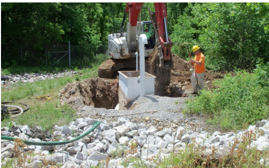
Tank Excavation
