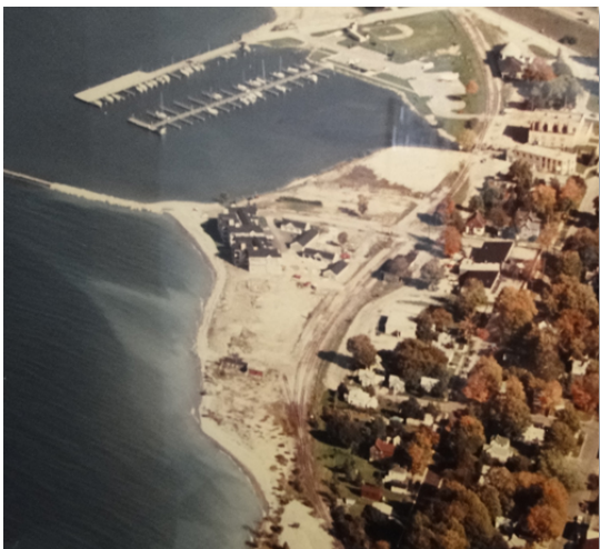
Figure 5. The site during redevelopment.
