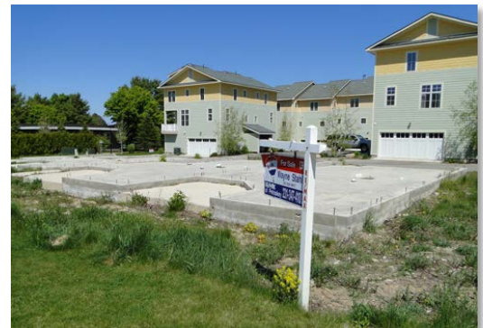
Figure 11. Water Street Condominiums – Phase III, during construction
