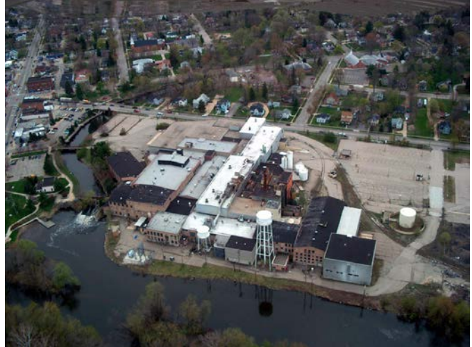
Aerial view of the mill in 2004.
