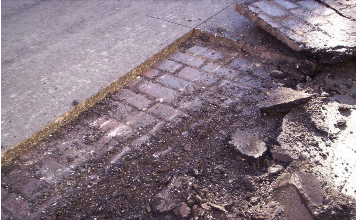
Photo 9: Taken east to west. Shows brick pavers (i.e., old pavement surface) beneath the asphalt surface at test pit #3 location that created elevated radiation surface screening count levels.
