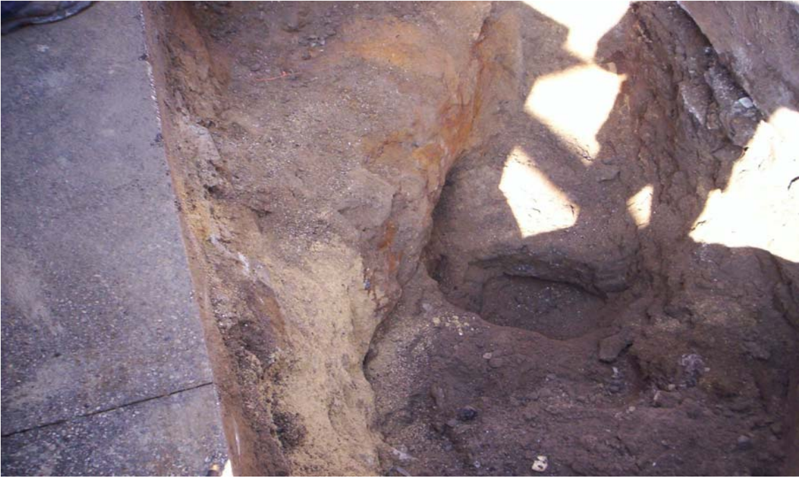
Photo 5: Taken south to north. Shows 24-inch gas main crossing test pit #1 location.
