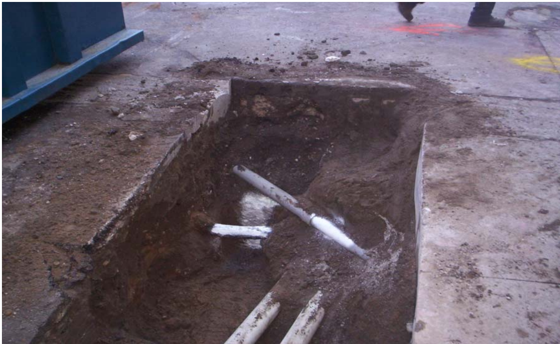
Photo 10: Taken south to north. Shows multiple utilities crossing test pit #4 location.
