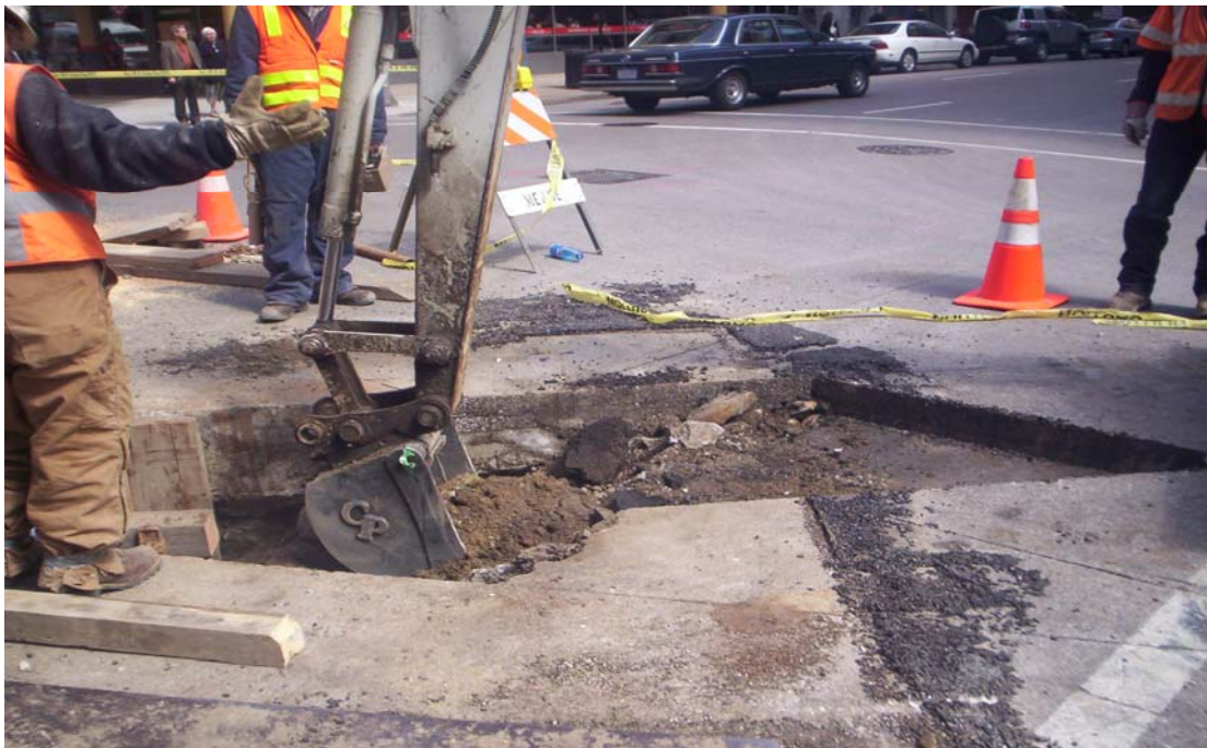
Photo 4: Taken west to east. Shows start of trench excavation heading southeast from the ComEd manhole on Ohio using a backhoe.
