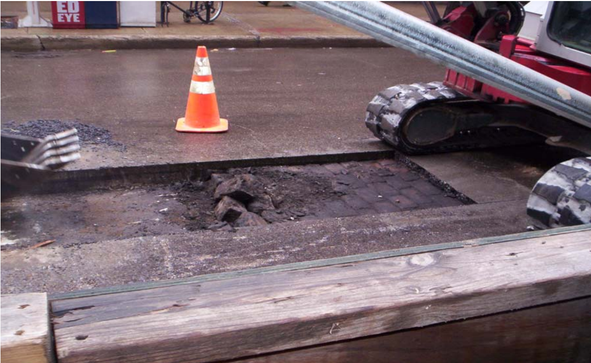
Photo 10: Taken west to east. Shows brick pavers (i.e., old pavement surface) beneath the asphalt surface along St. Clair that yielded radiation count levels above background readings.
