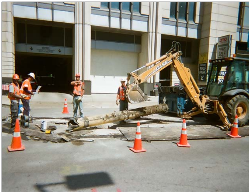
Photo 8: Taken south to north. Removal of out-of-service natural gas main encountered during excavation after cutting into sections.
