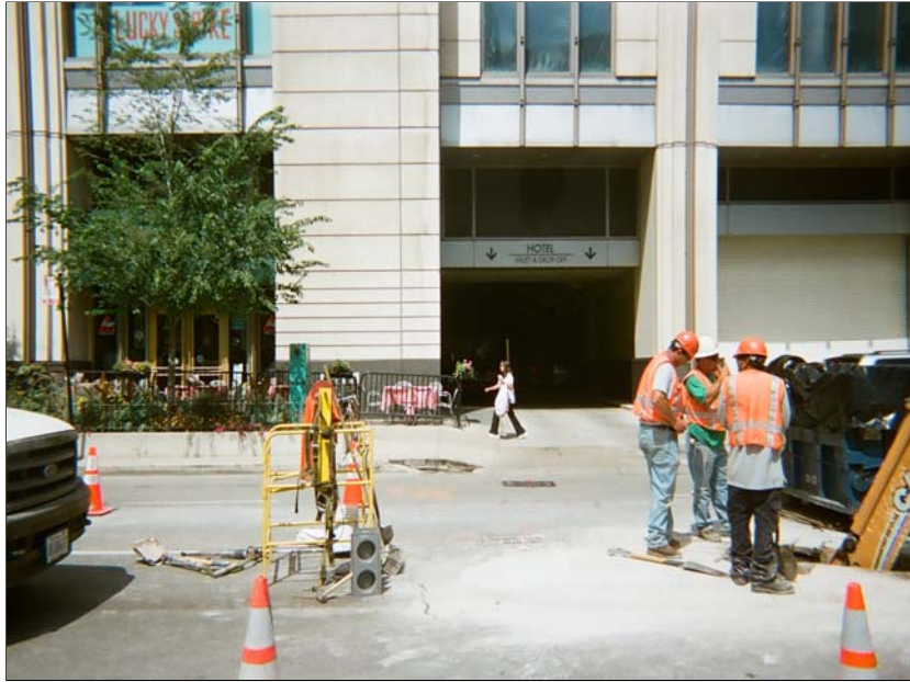
Photo 3: Taken south to north. Manhole starting point for trench on Illinois Street at beginning of excavation.
