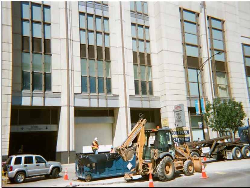
Photo 7: Taken south to north. Composite soil sample being collected from full roll-off box for radiation analysis in 20-ml vial after homogenization.
