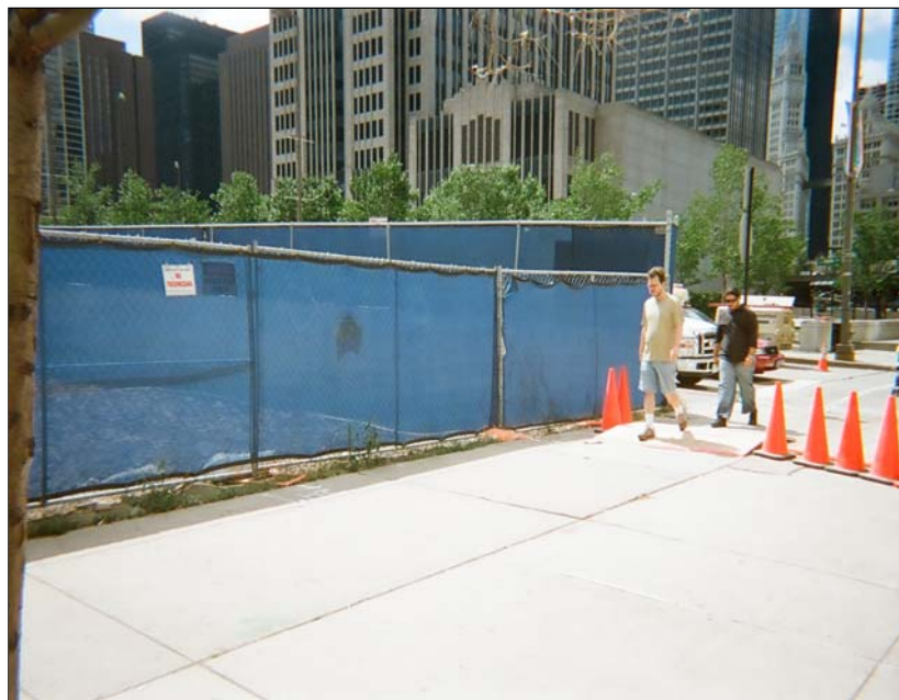
Photo 2: Taken east to west. Conduit tie-in location at property line across sidewalk prior to beginning excavation. Site currently undergoing construction.
