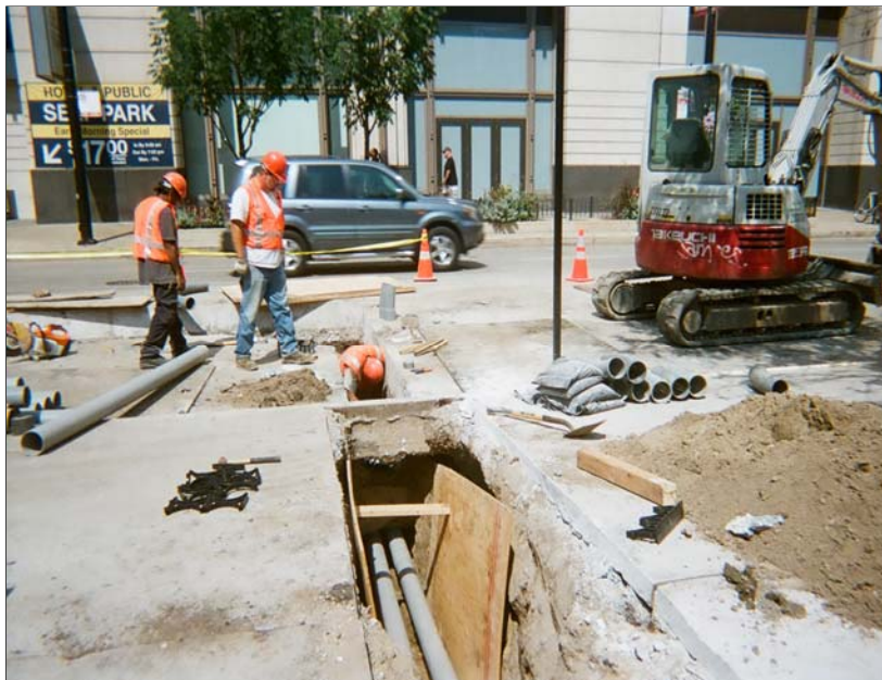
Photo 10: Taken south to north. Installation of conduit pipes in north to south trench section at the completion of excavation and radiation monitoring.
