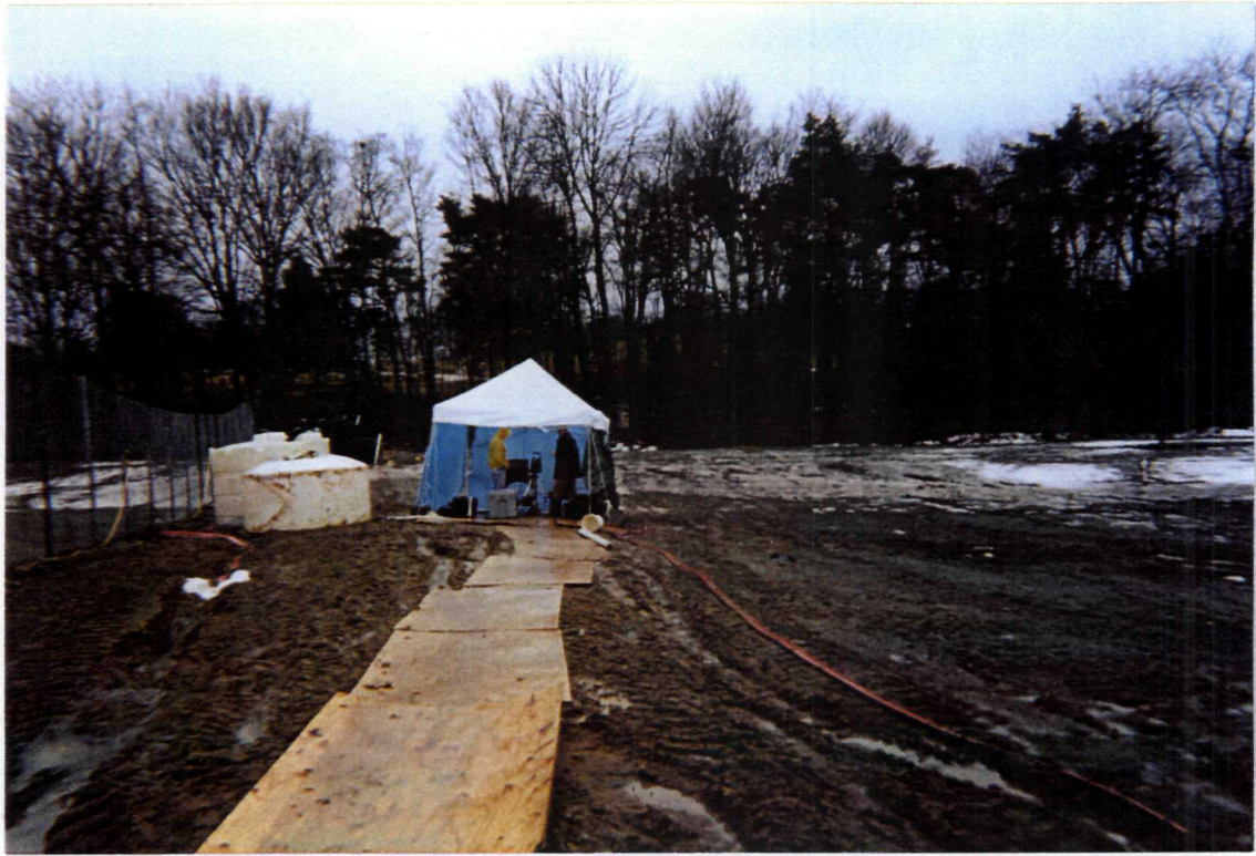
Photograph No. 1 Orientation: South
