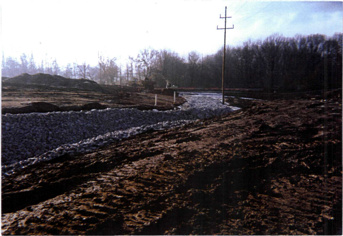
Photograph No. 1 Orientation: Southeast Description: WRS working on site perimeter drainage ditch
