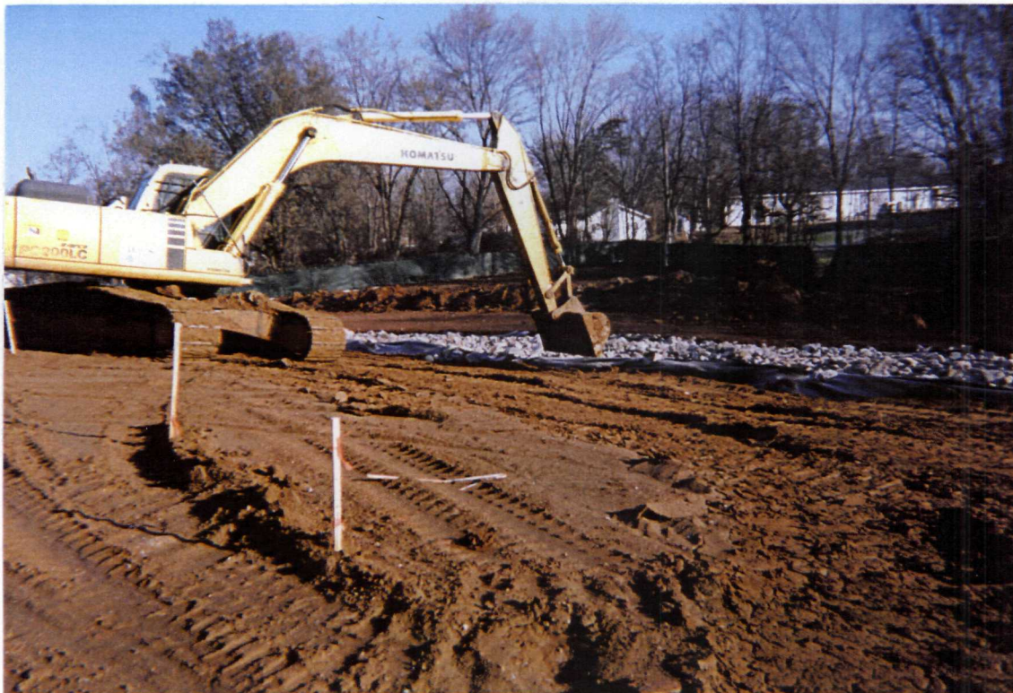
Photograph No. 1 Orientation: Southeast Description: WRS working on site perimeter drainage ditch
