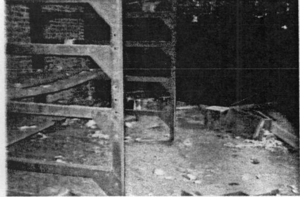
Building #12 – Sample B12-39
