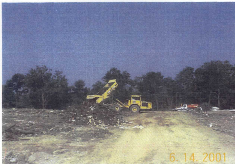
Photo 6. Waste placement near the northwest corner of the landfill. Decon pad is shown at right background.
