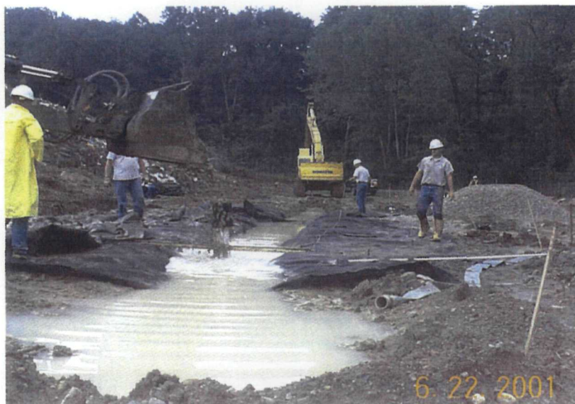
Photo 7. Construction of Interceptor Trench #1.
