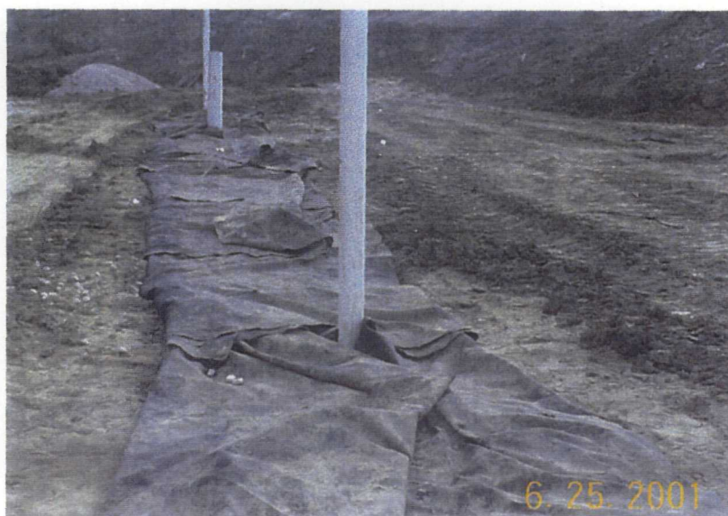
Photo 8. Construction of Interceptor Trench #1.
