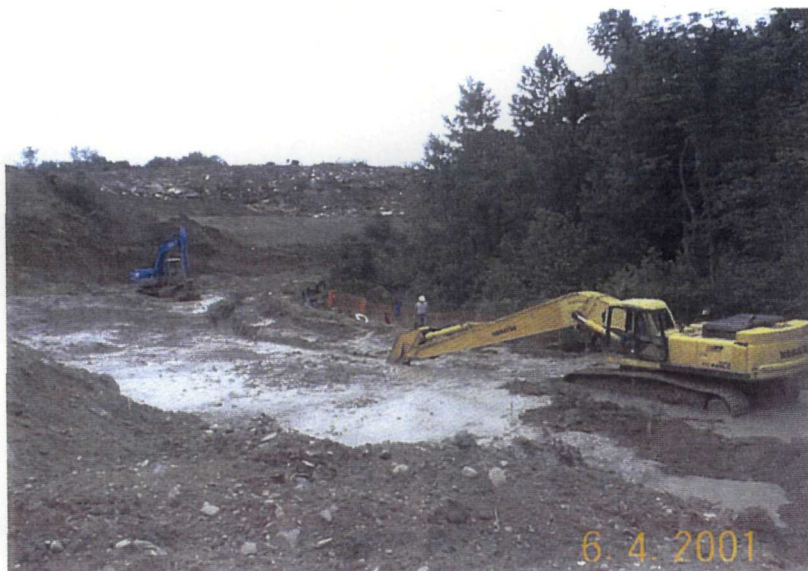
Photo 2. Construction of Slurry Wall near Station 7+00.
