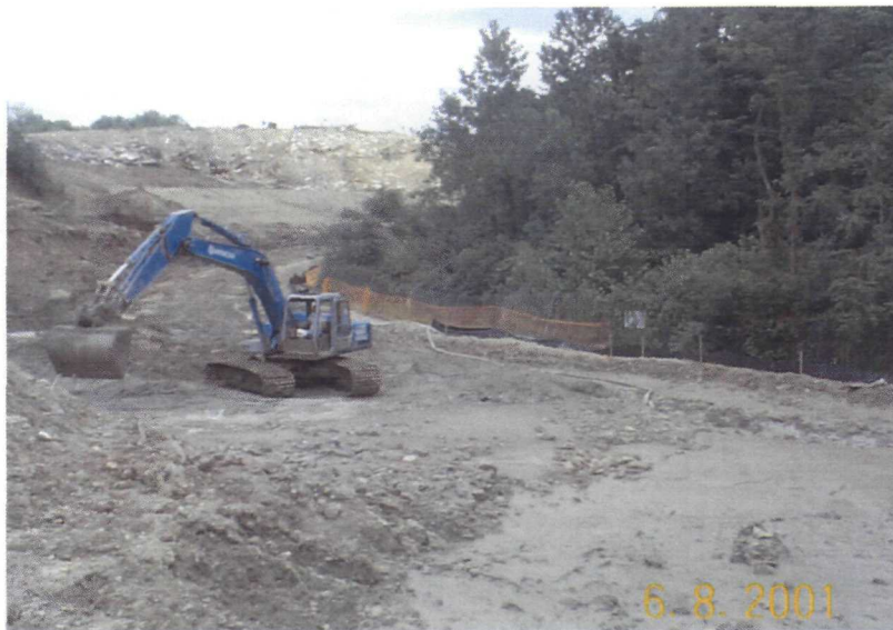
Photo 3 Slurry dry-out area shown at right foreground.
