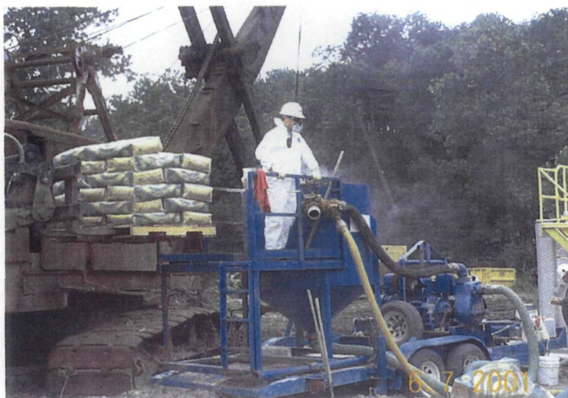
Photo 5. Pug mill for bentonite-water slurry mixture.
