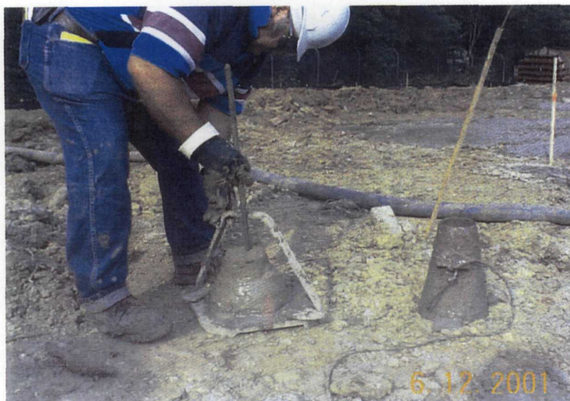
Photo 4. Field QA/QC testing (slump) of slurry-soil mixture.
