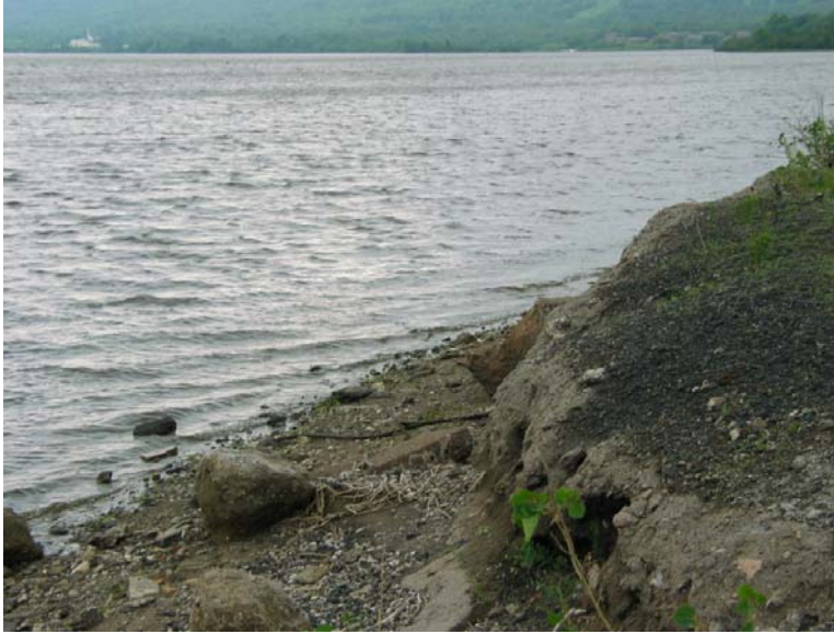
Viewed here is erosion observed at the southern tip of the 59 th Avenue peninsula.
