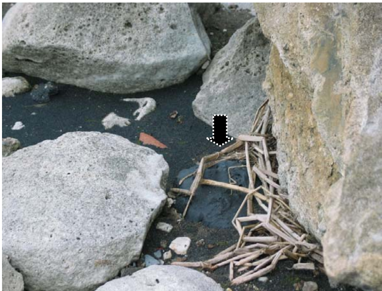
This tar was observed in the same general location that the erosion was noted. The tar and erosion location are approximated on Figure 7 as Area F 3.
