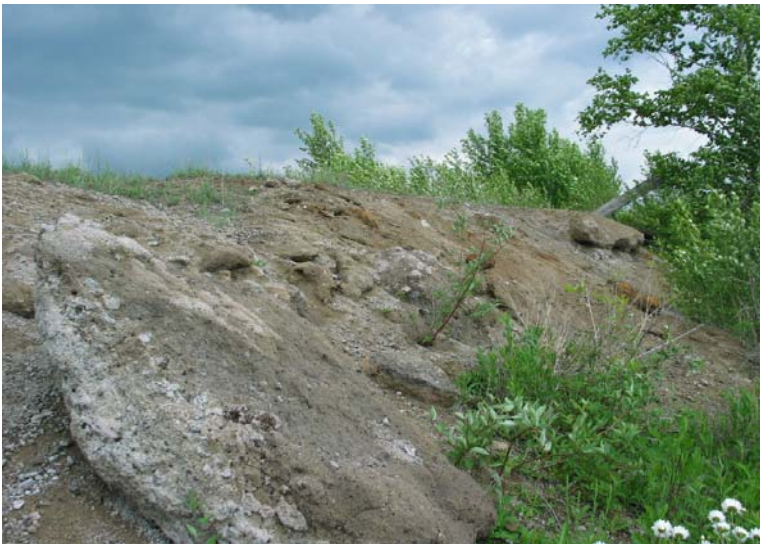
Erosion along the west shore of the 59 th Avenue peninsula was observed. The location was marked using GPS and is shown as Area F 2 on Figure 7
