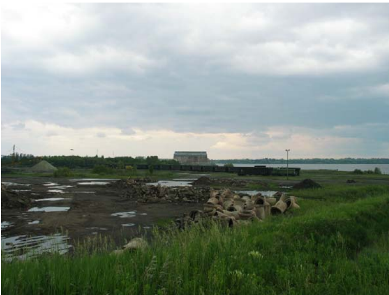
Photographed to the left is the concrete recycling operation as seen on June 25, 2003 from top of berm looking east.
