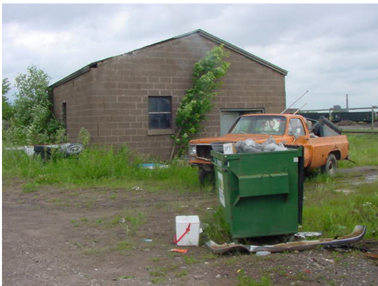
Residual Contamination is present under this pump house in Area D.
