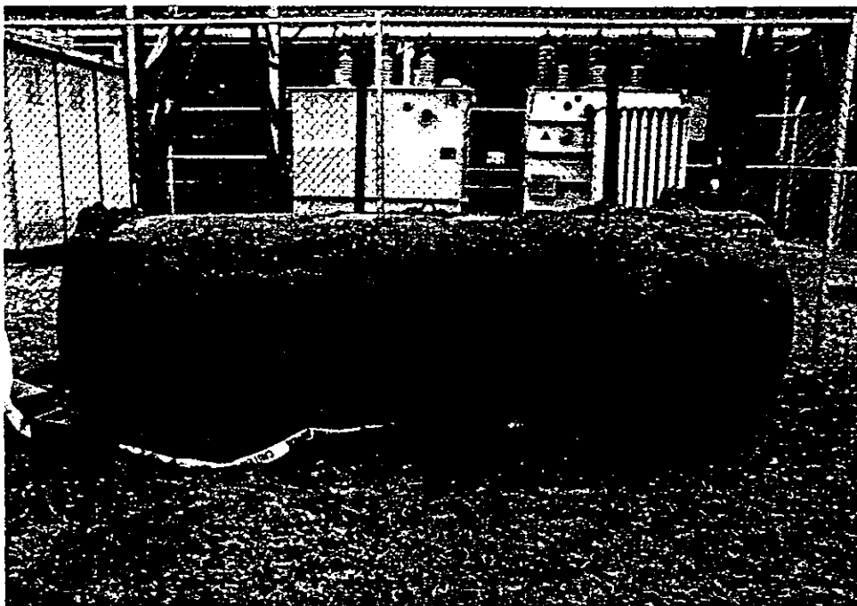
UST No. 6 Staged for final cleanout and inspection
