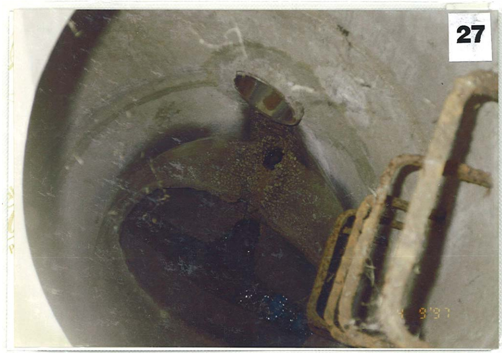
Figure 1. Suggested 6-inch former process waste sewer line inlet to 15-inch storm sewer. (From Appendix I – Baseline Assessment Site Inspection Photographs, Baseline Environmental Assessment, Payne Firm, 1997).
