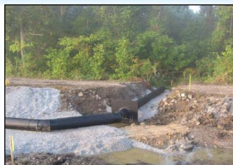
3 INSTALLED HDPE PIPE IN ROAD CROSSING AREA AND INTO ORIGINAL DRAINAGE DITCH.
