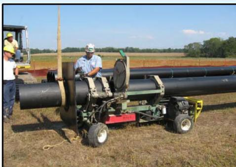
2 FUSING HDPE DRAINAGE PIPE PRIOR TO INSTALLATION
