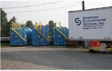
RECEIVED FRAC TANKS IN PREPARATION OF MOD-U-TANK DECOMMISSIONING
