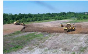
CONTINUING TO PLACE, GRADE AND COMPACT SUB GRADE SOIL IN THE FORMER PROCESS AREA SURFACE COVER
