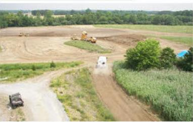
**WATERING ROADS FOR DUST CONTROL, FINISH GRADING WETLANDS AND STOCKPILING VEGETATIVE SOIL**
