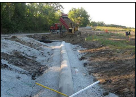
4 BACKFILLING HDPE DRAINAGE PIPE WITH GRAVEL.
