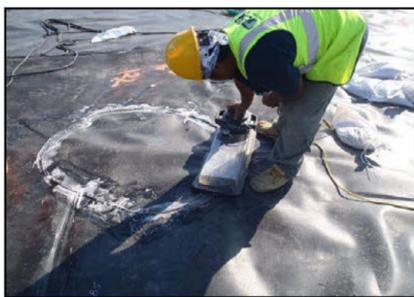
1 VACUUM TEST ON A PATCH ON THE HDPE LINER.
