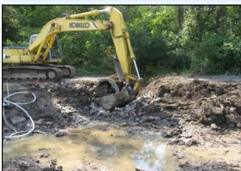
1 REMOVING EXISTING 36 INCH CONCRETE PIPE FROM ROAD CROSSING AREA.
