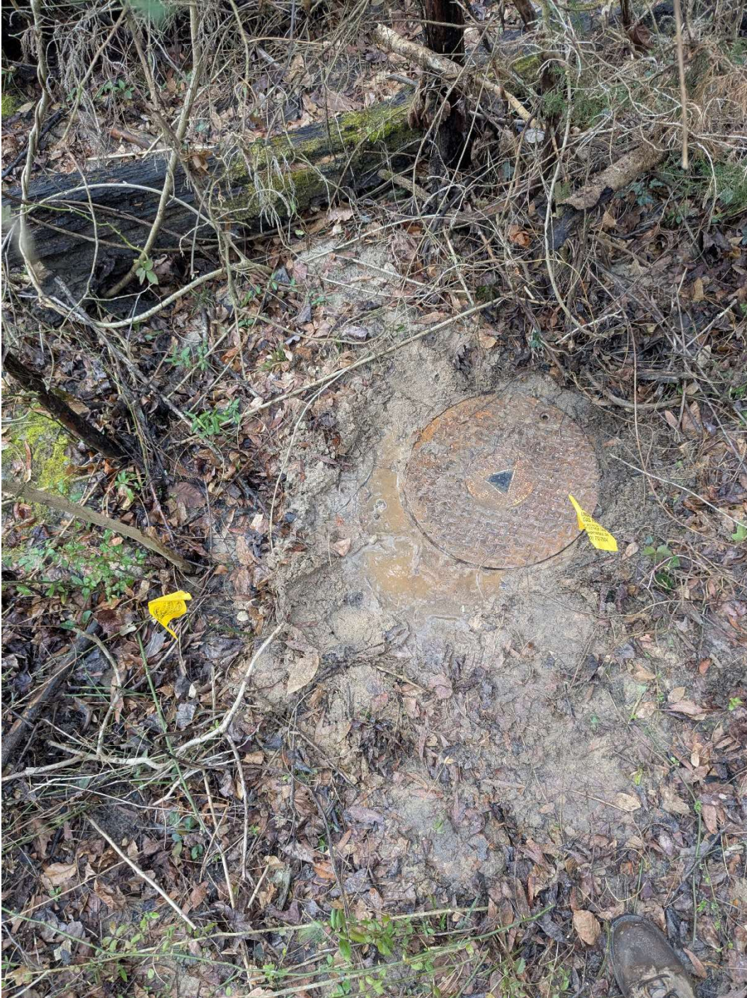
FIGURE C7: MW-2 Well manhole covering, 1/4" of sediment cleared from well cover
