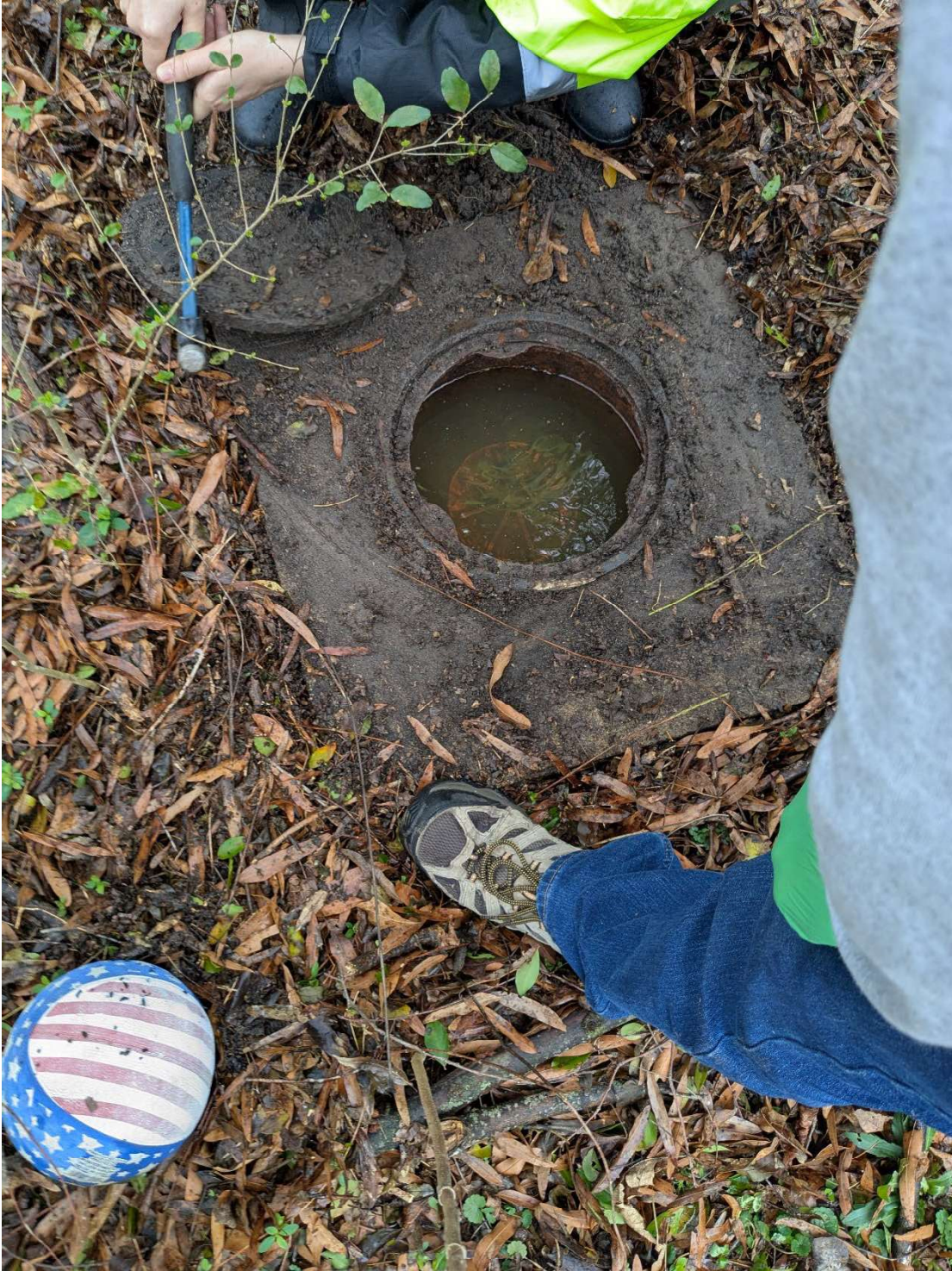
FIGURE C5 : MW-15 Inside housing flooded. Well was able to be sampled, but casing infiltration required constant pumping
