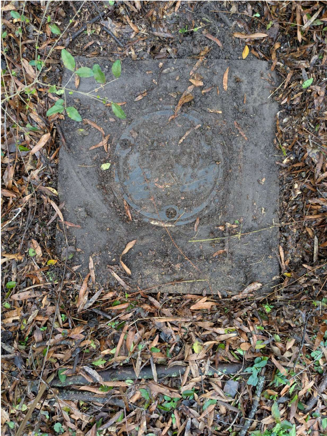
FIGURE C4 : MW-15 Well pad after clearing debris and sediment
