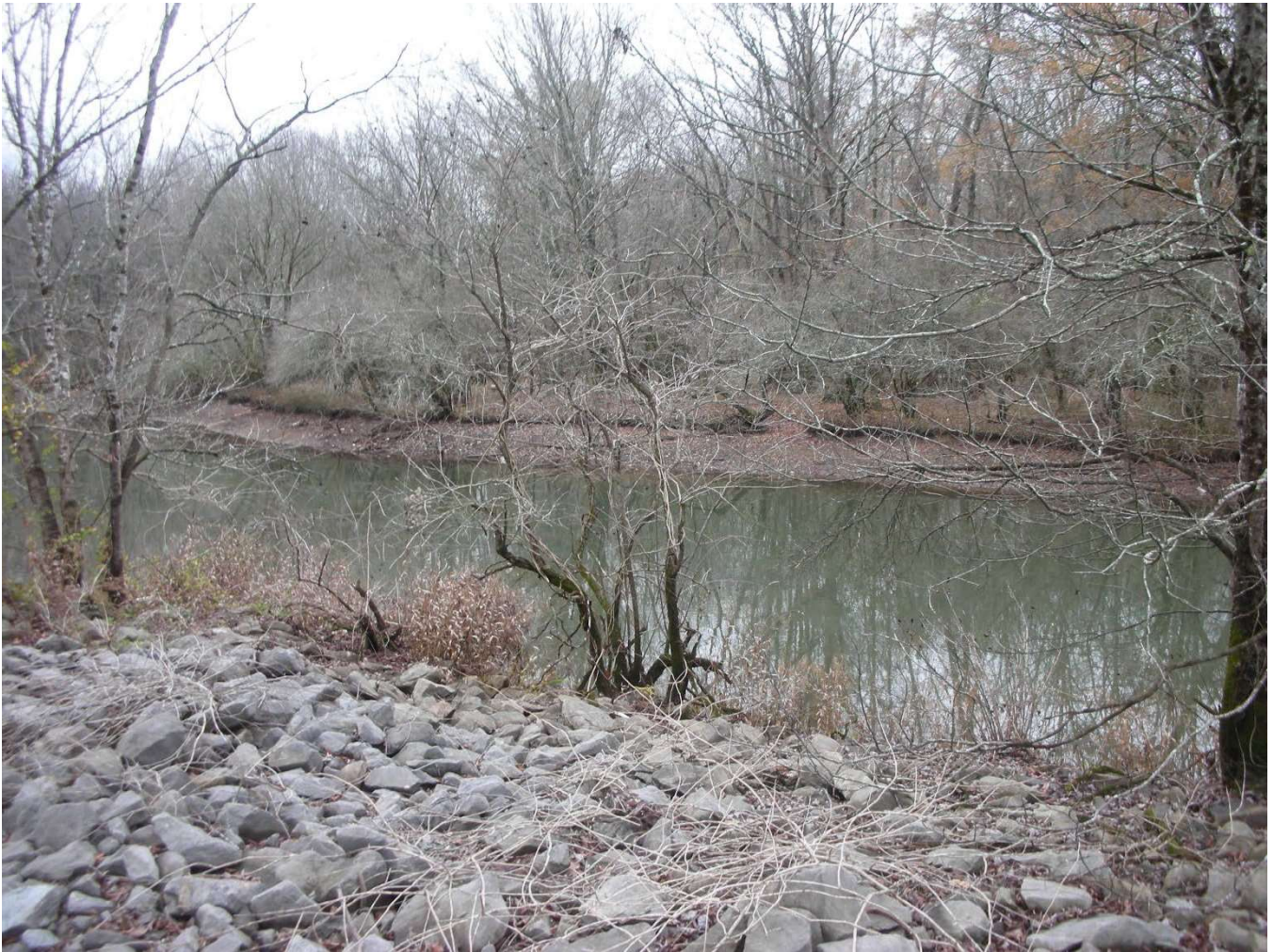
Photograph F-6: Stream levels and riprap stabilization along Reach A
