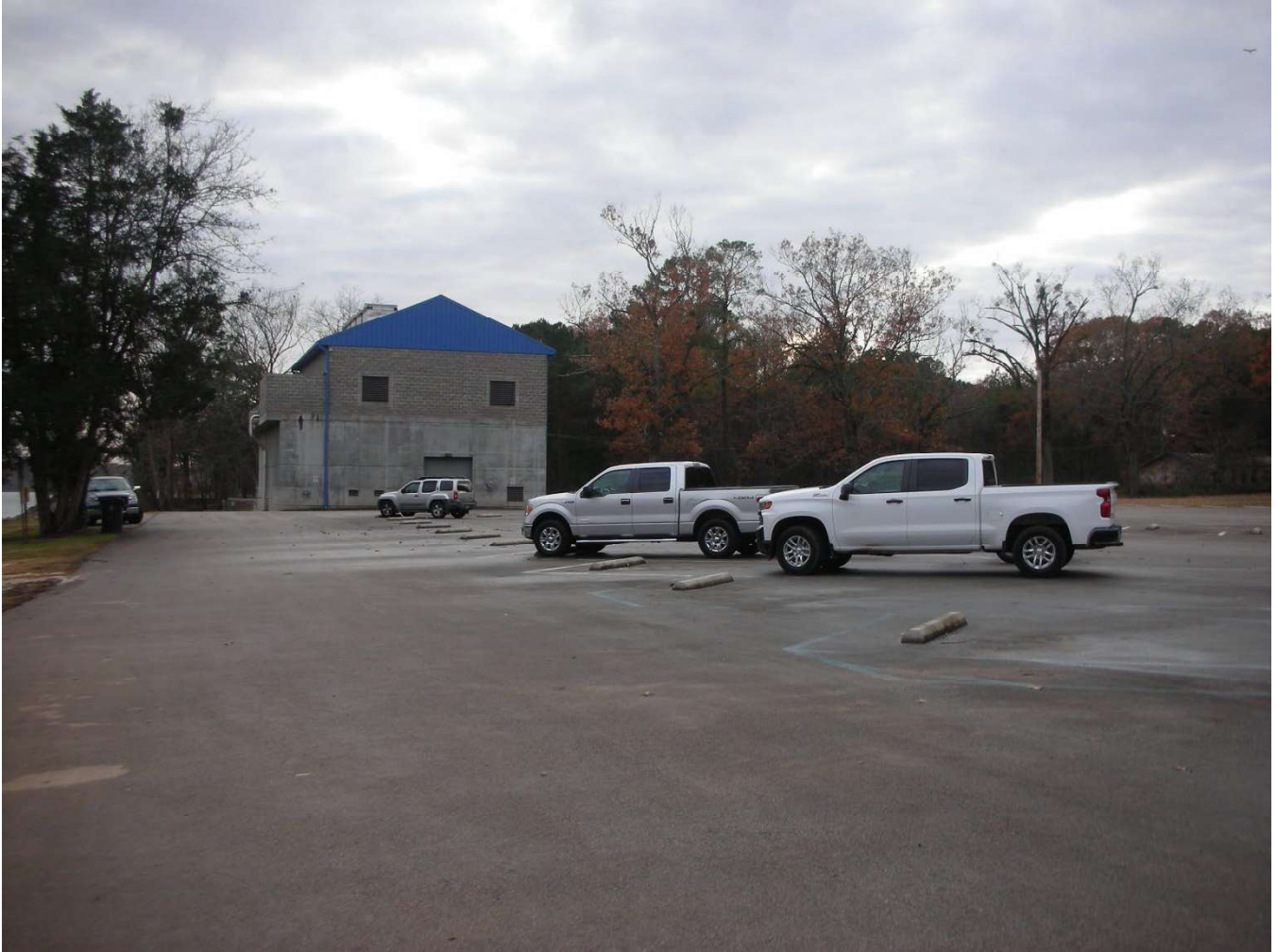
Photograph F-1: Triana Water Intake facility and public boat launch
