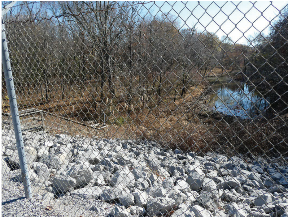
Surface water sampling location on the southeast end of Airco landfill
