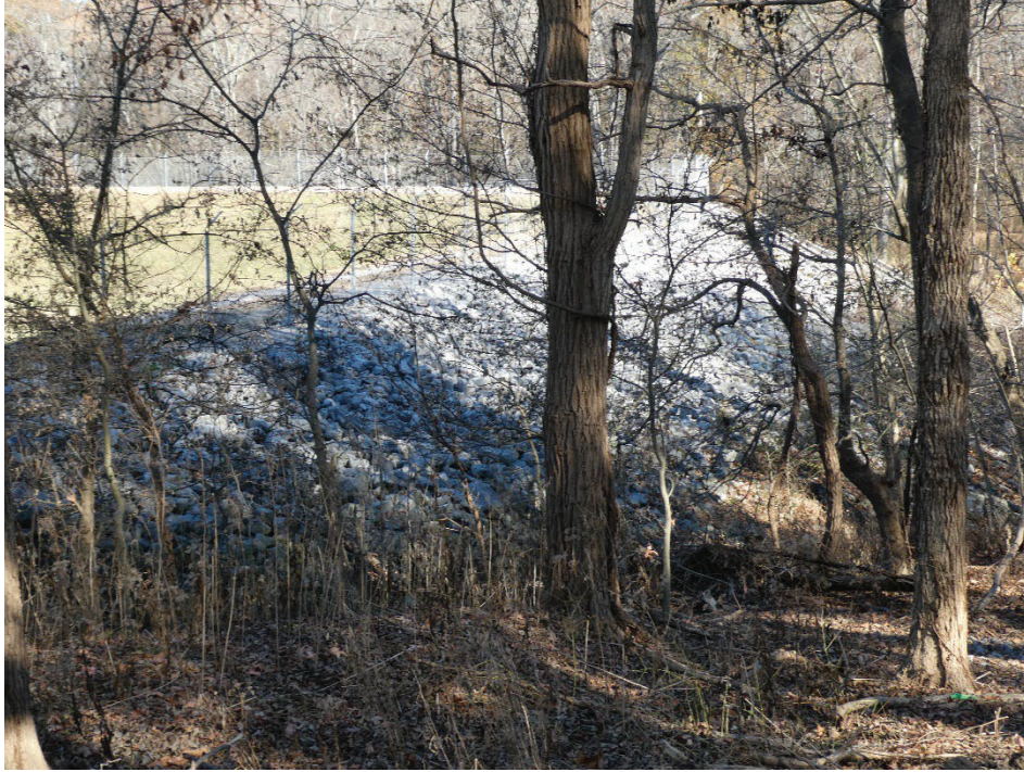
Flood protection dike on the southeast end of Airco landfill
