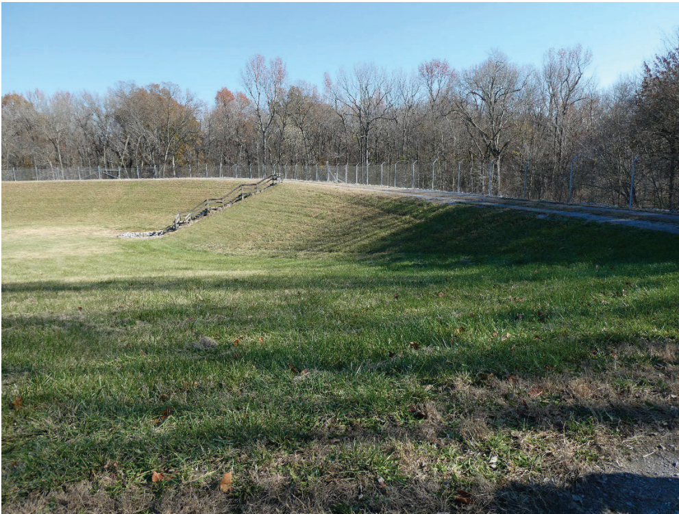
Airco landfill looking northeast
