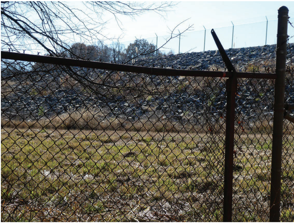
Flood protection dike northeastern side of Airco landfill
