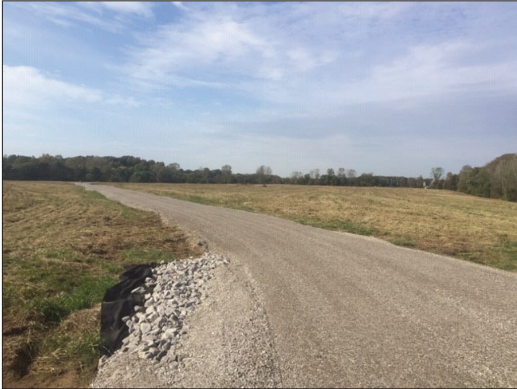
Vegetated cap and gravel road at the West Sector disposal area.
