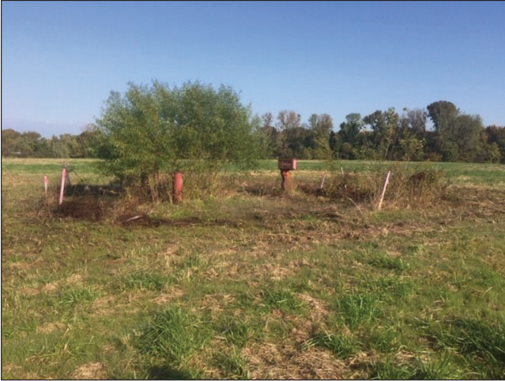
Cluster of wells located on the vegetated cap of the East Sector disposal area.
