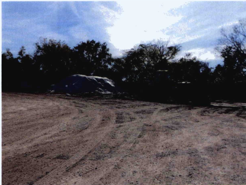
COJ staging area for soil excavations
