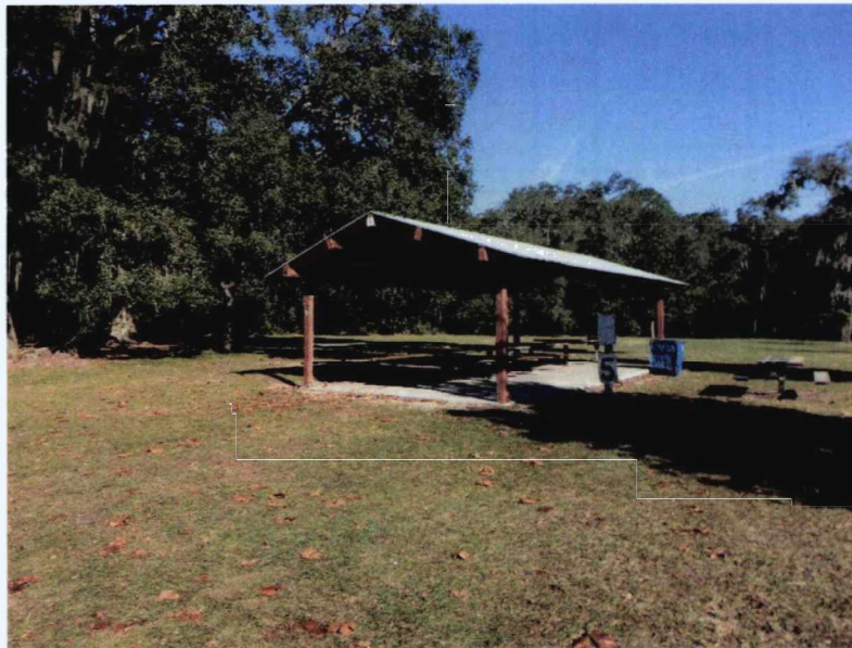
Lonnie C. Miller Sr. Park picnic shelter
