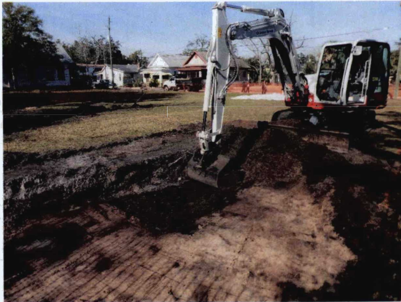
Active remediation in a neighborhood on site
