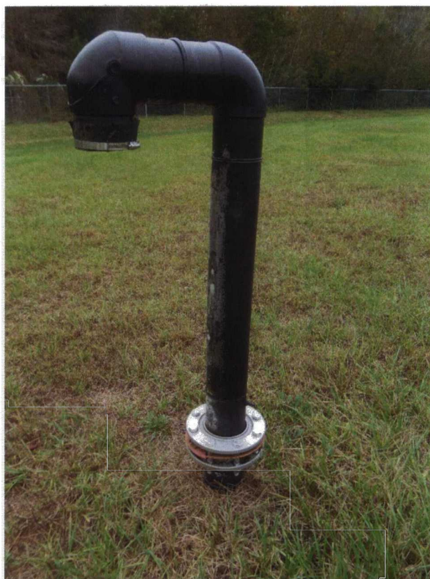
Gas vent on vegetated capped area
