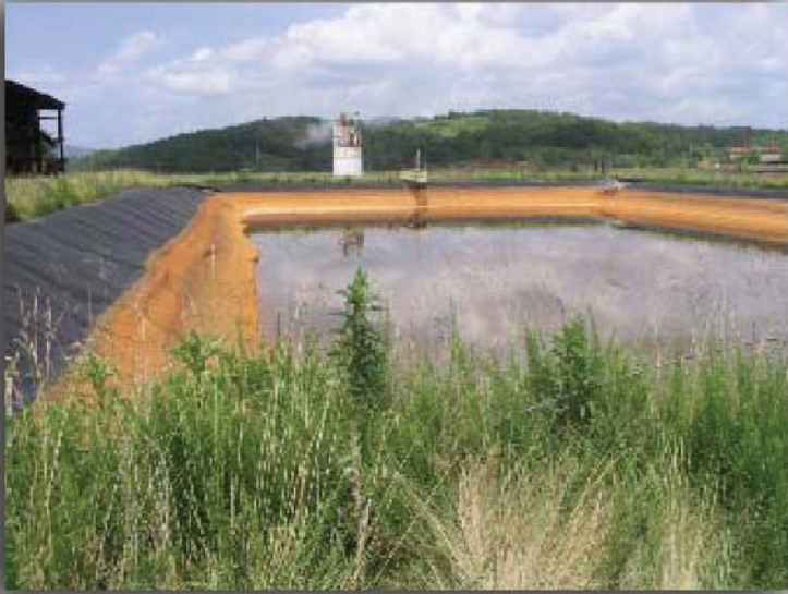
Surface impoundment for Cantrell Flats Wastewater Treatment Plant
