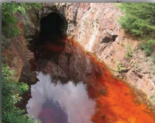
Former diversion tunnel outfall in the Davis Mill Creek watershed
