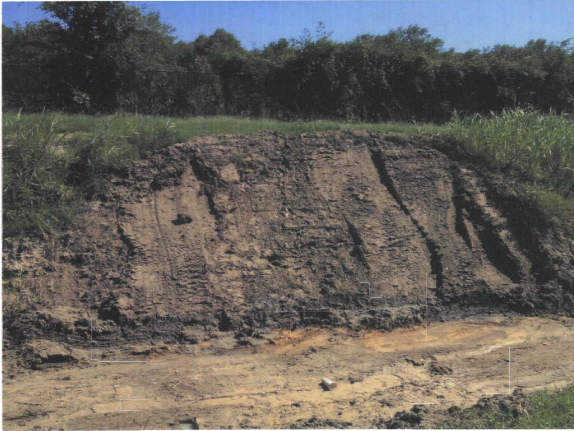
Photo #1: Repaired failure of the existing pond berm between the southern end of Ditchline 2 and the existing pond.
