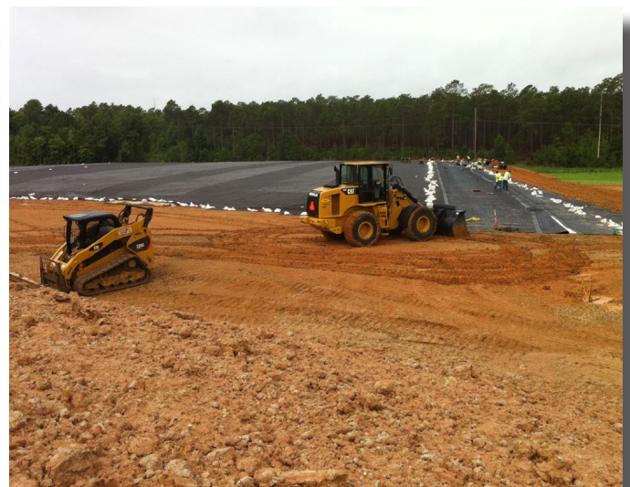
The site's impoundment area under construction, 2012.
