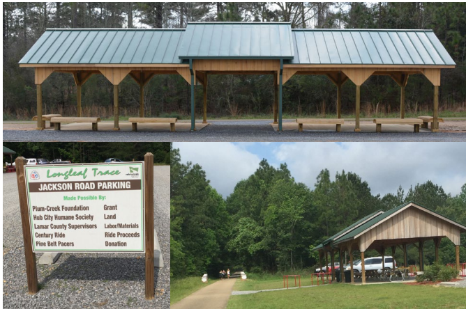
Views of the Longleaf Trace Trail pavilion and parking area, located next to the Fields of Barktopia.
