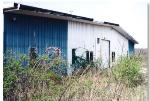
Figure 2. Former Transicoil facility prior to site cleanup.
