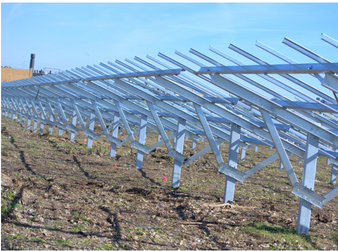
Mounting rack installation.
