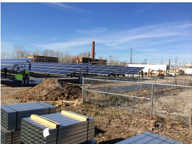
Solar panel installation.
