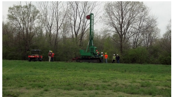
Field testing of pile installation.
