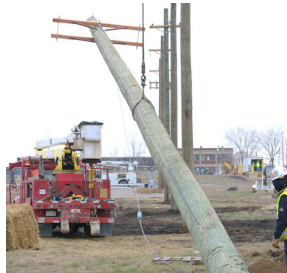
Utility pole installation.
