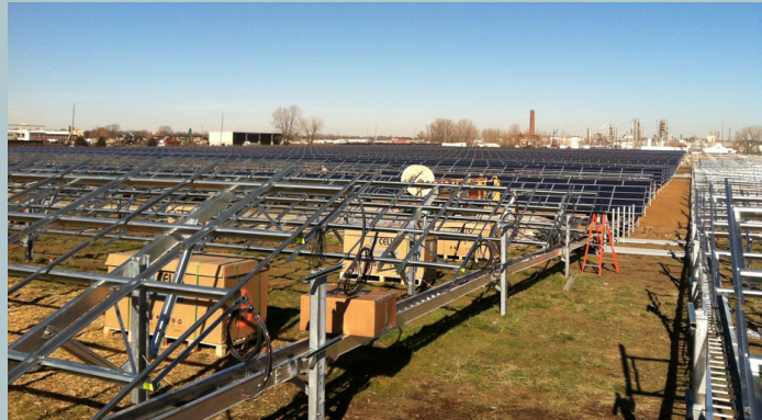
Panel mounting system installed at Maywood Solar Farm. The system includes an innovative above-ground wire management approach.
