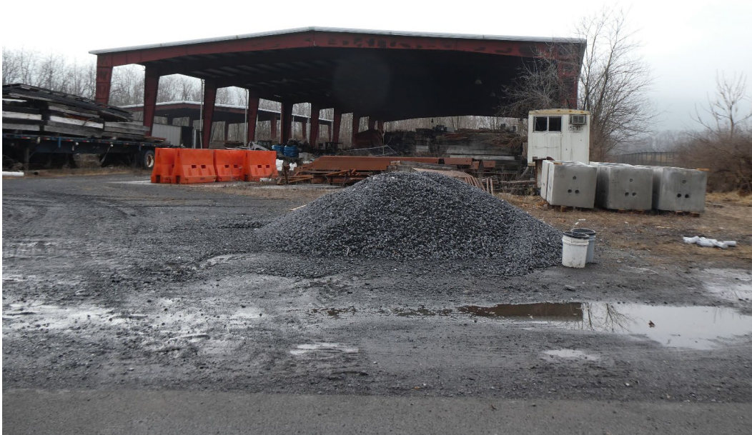
Storage shed in Zone 1
