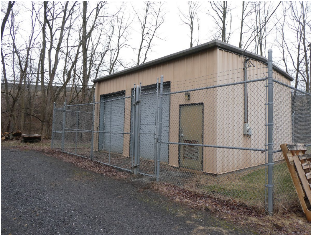
Groundwater extraction and treatment building in Zone 2
