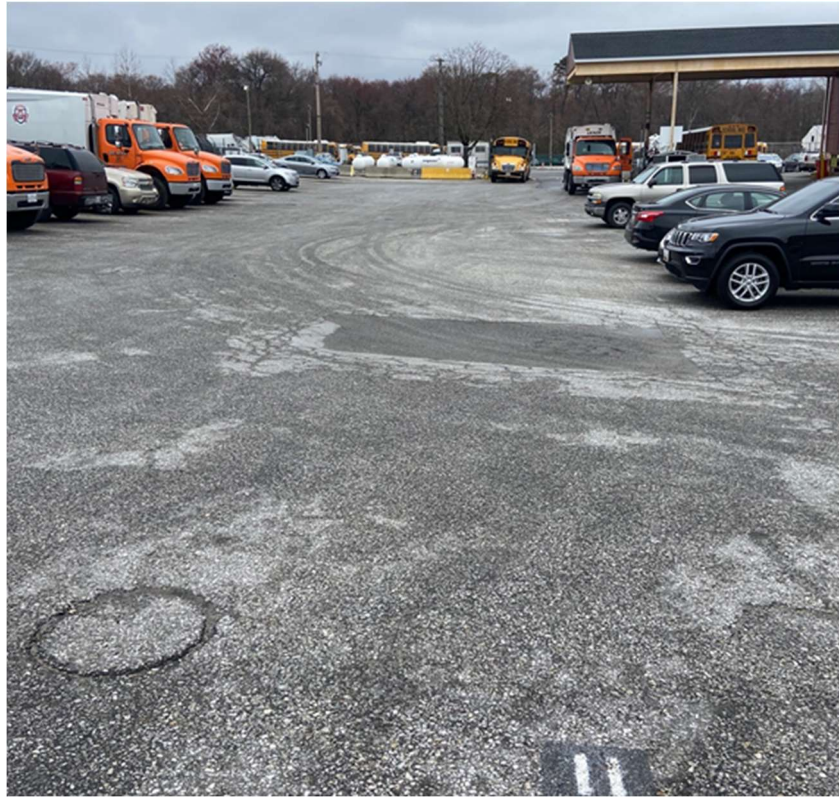
Asphalt cap in Treatment Yard – 3/13/2023
