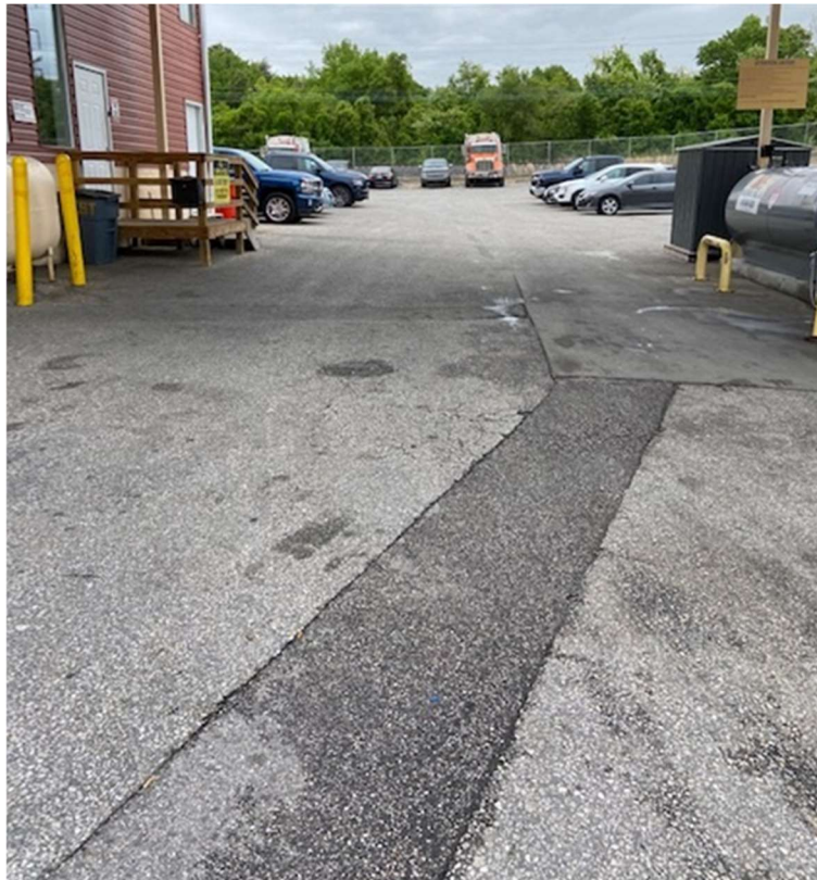
Asphalt cap at Treatment Yard – 5/2/2023
