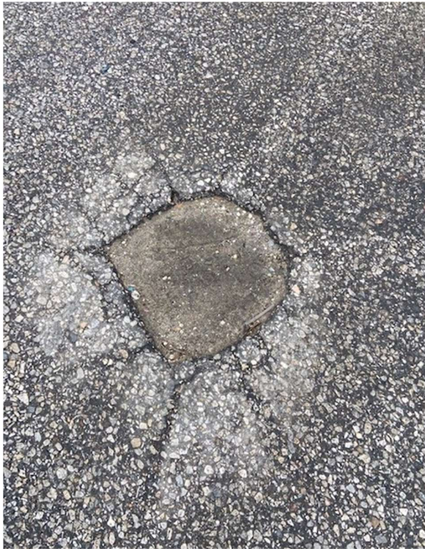
Small hole where propane tank was removed in Treatment Yard – 3/13/2023
