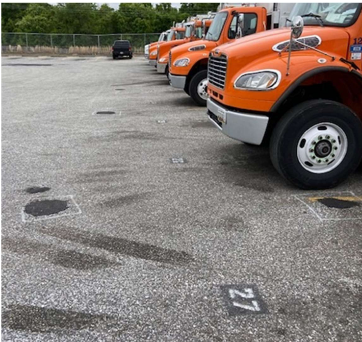
Asphalt repair where propane tank was removed in Treatment Yard - 5/2/2023
