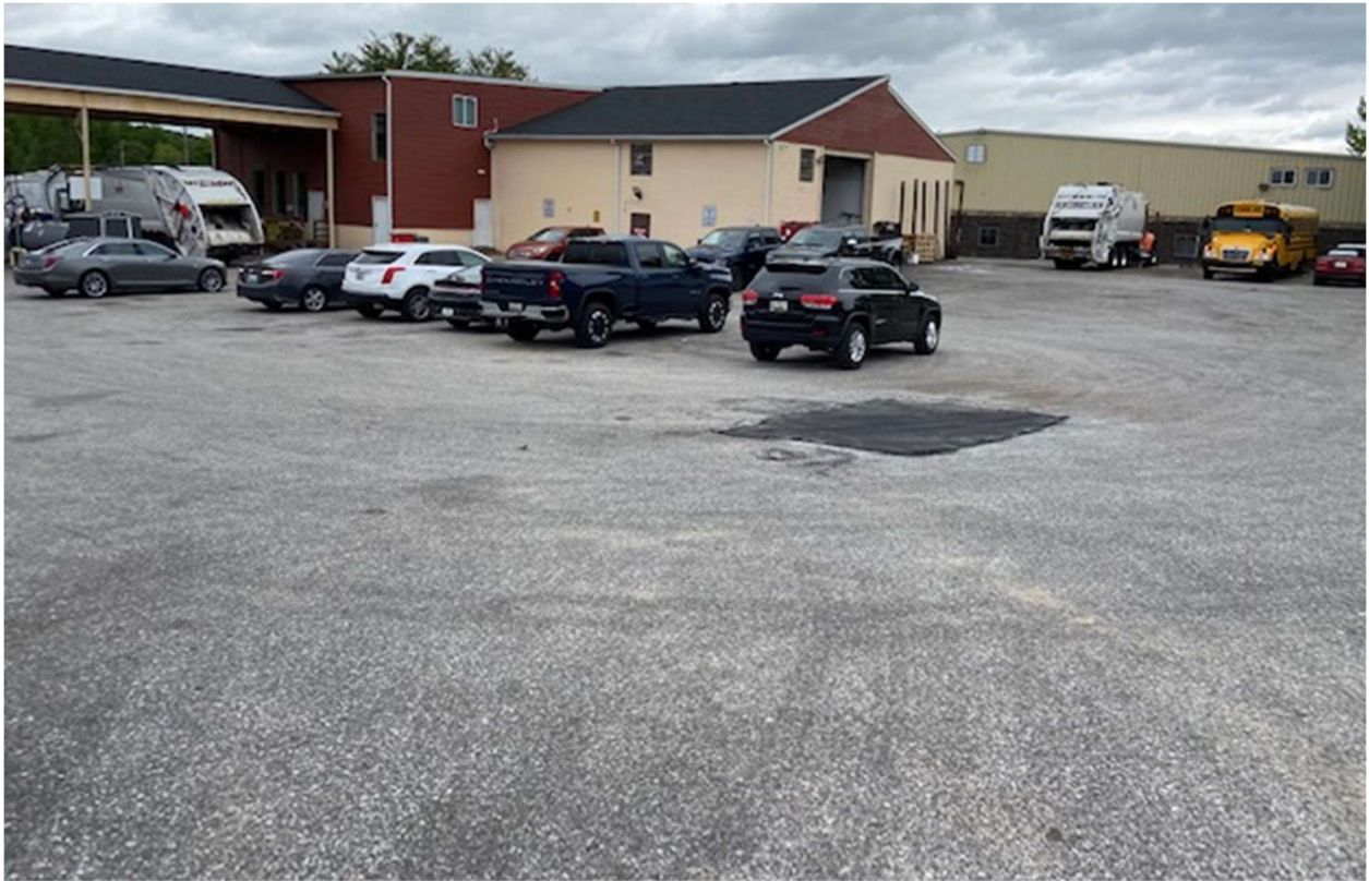
Asphalt cap at Treatment Yard – 5/2/2023
