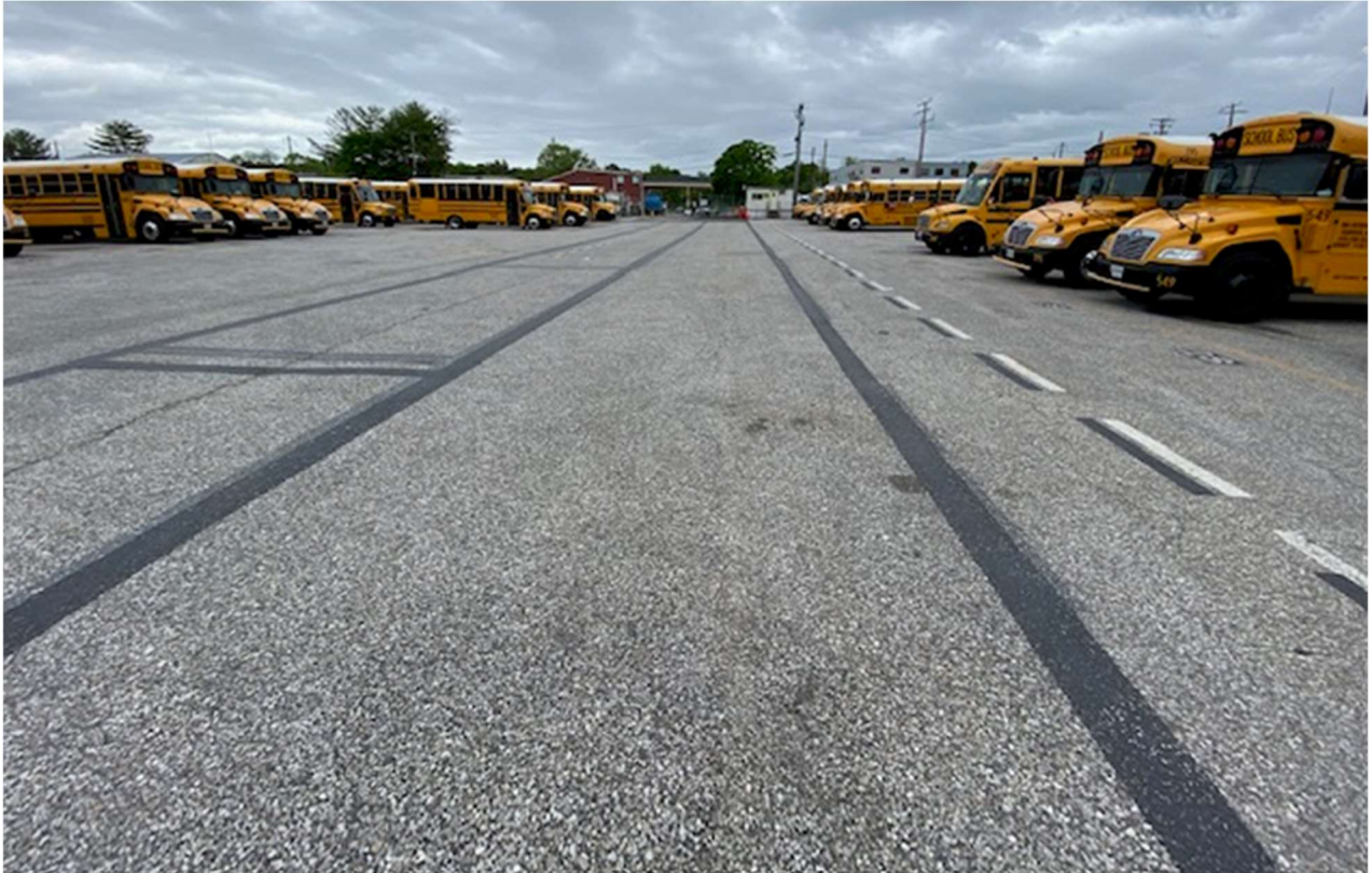
Storage yard asphalt cap - 5/2/2023
