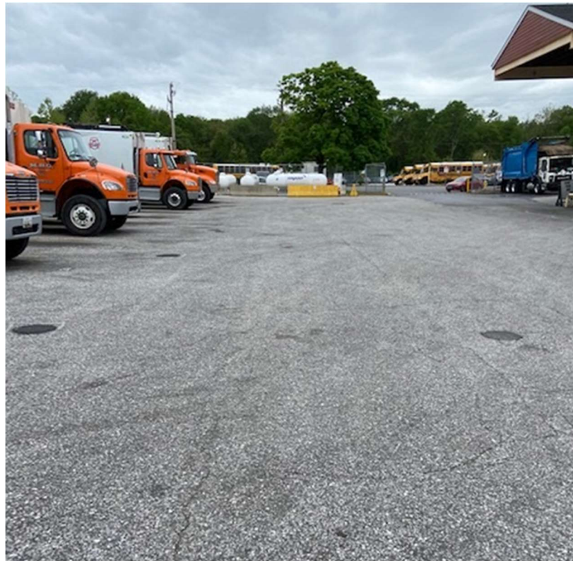
Asphalt cap in Treatment Yard after repairs were made to cap - 5/2/2023
