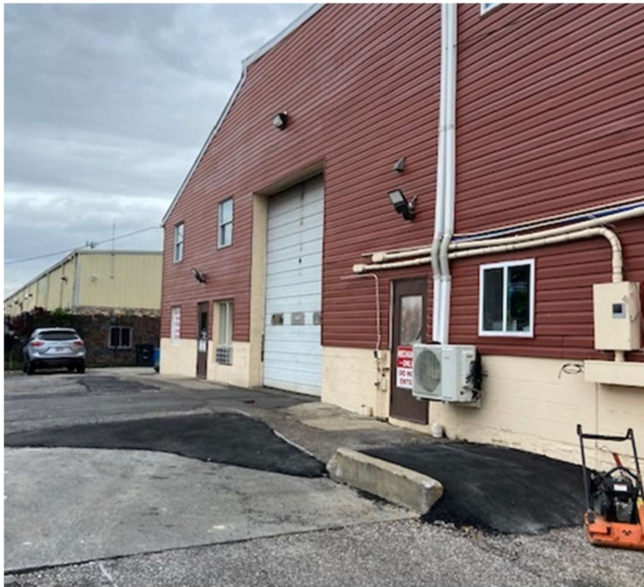
Asphalt repair around former treatment building - 5/2/2023
