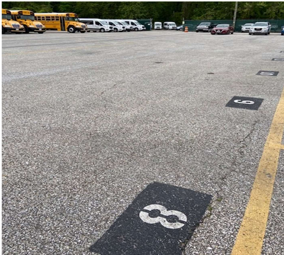
Storage yard asphalt cap - 5/2/2023
