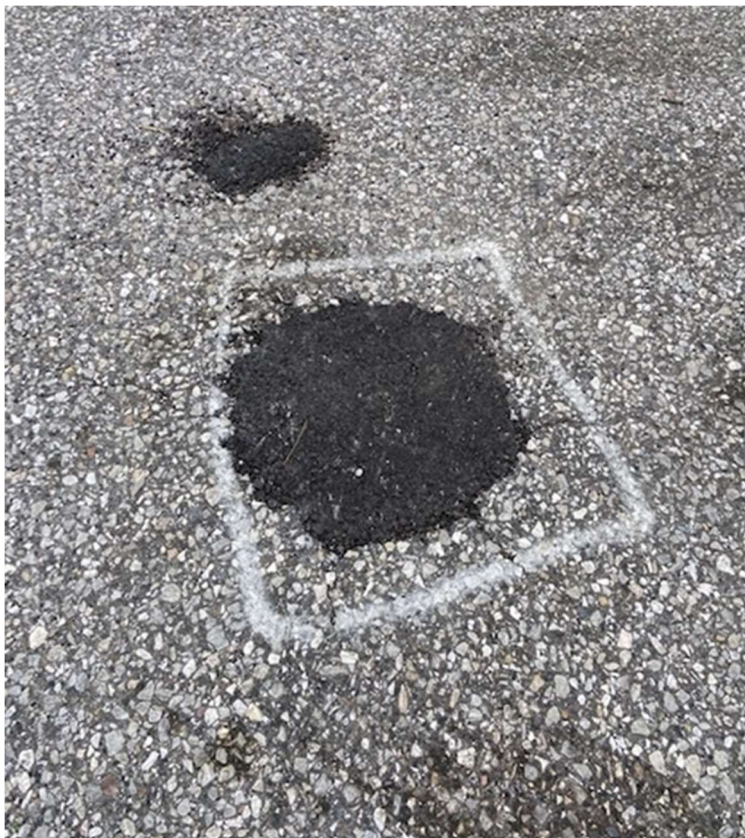
Asphalt repair where propane tank was removed in Treatment Yard - 5/2/2023
