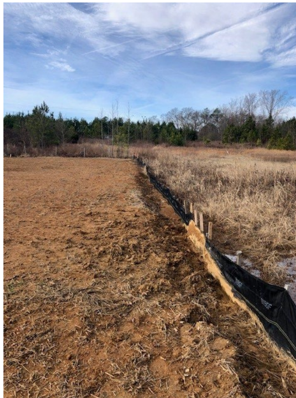
View of northern boundary of 1320 Bellwood Road, facing west.
