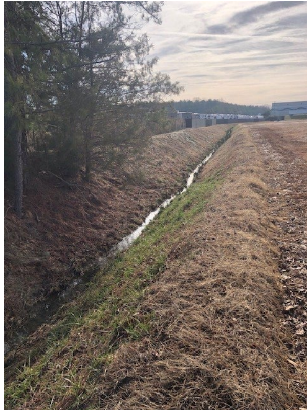
View of drainage ditch located on eastern boundary of 1320 Bellwood Road, facing south.
