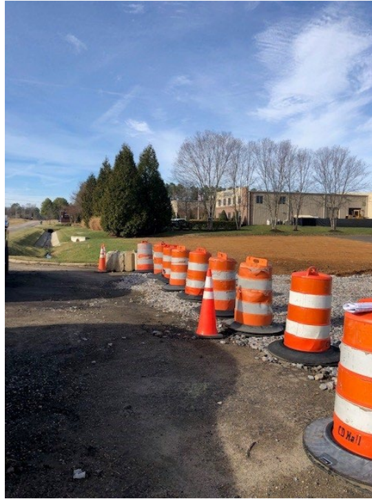
Entrance to 1320 Bellwood Road, facing southwest (parcel 7986770448)
