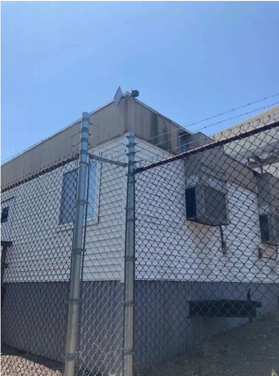
Office Trailer with 24 hour surveillance
