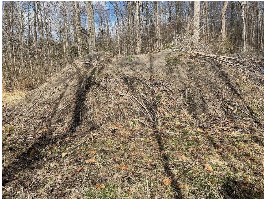
PHOTOGRAPH 05: Stockpiles of mixed crushed limestone and biosolids. Old silt fencing around piles, as well as a tarp (not pictured). Silt fencing and tarp to be removed. Stockpiles to be removed and used elsewhere.
