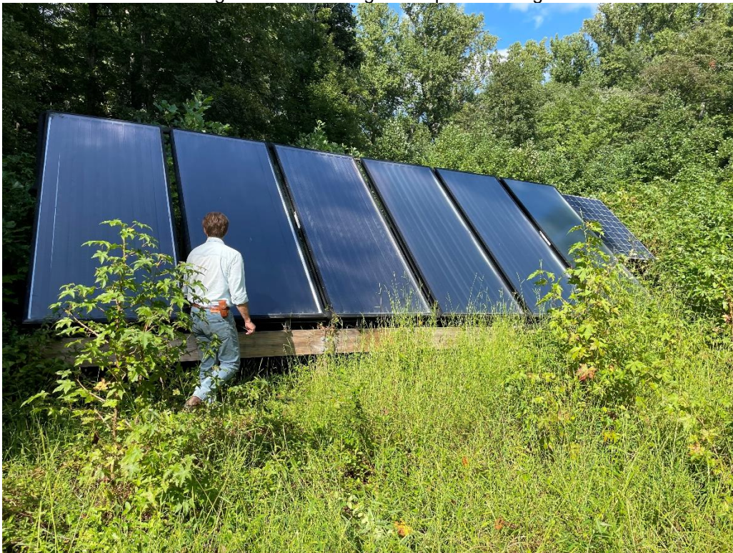
PHOTOGRAPH 04: Solar panels to heat water for circulation through selected upgradient trench pits (See Figure 1). There were no signs of damage or tampering on this system at time of inspection. Vegetation in clearing will require clearing.
