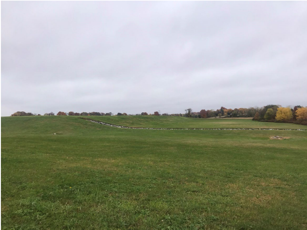
Stormwater drainage off landfill cap to wetland
