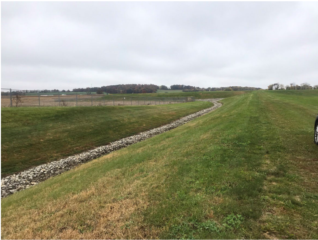
Stormwater drainage system surrounding the cap and fence
