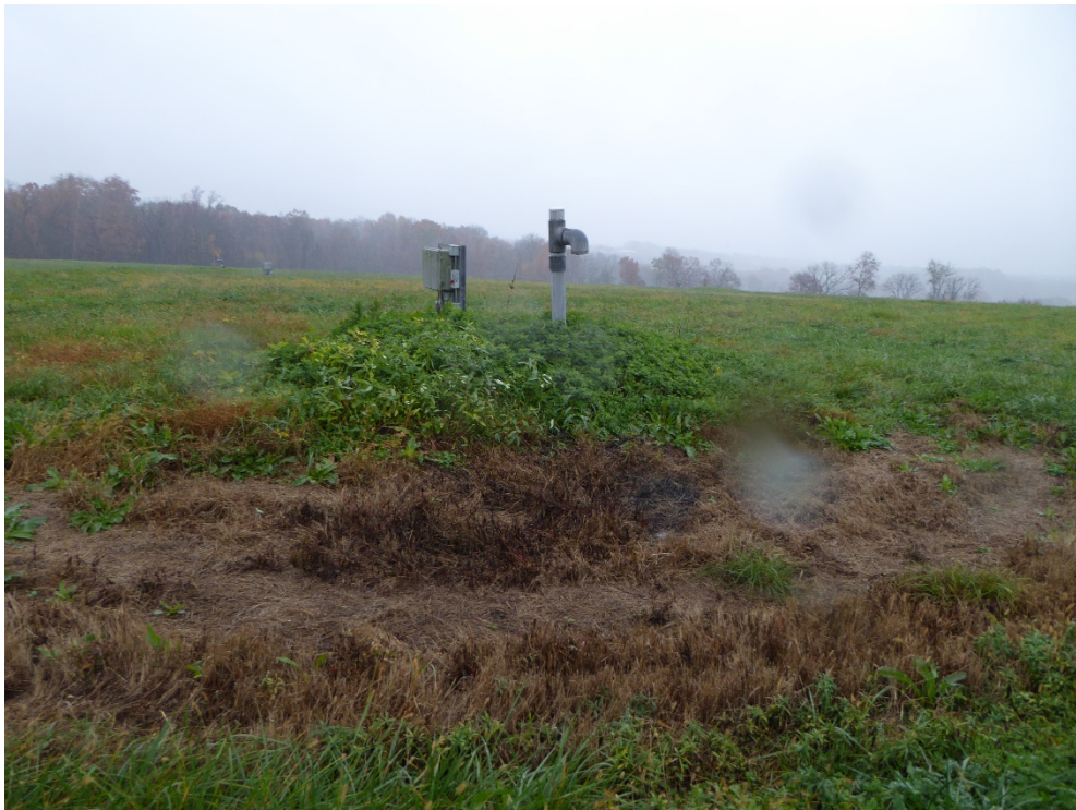
Photo 5: Landfill gas vent B-1
