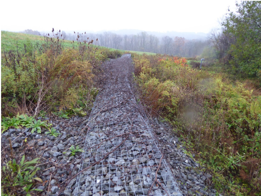
Photo 8: Gabion wall near GMP-2
