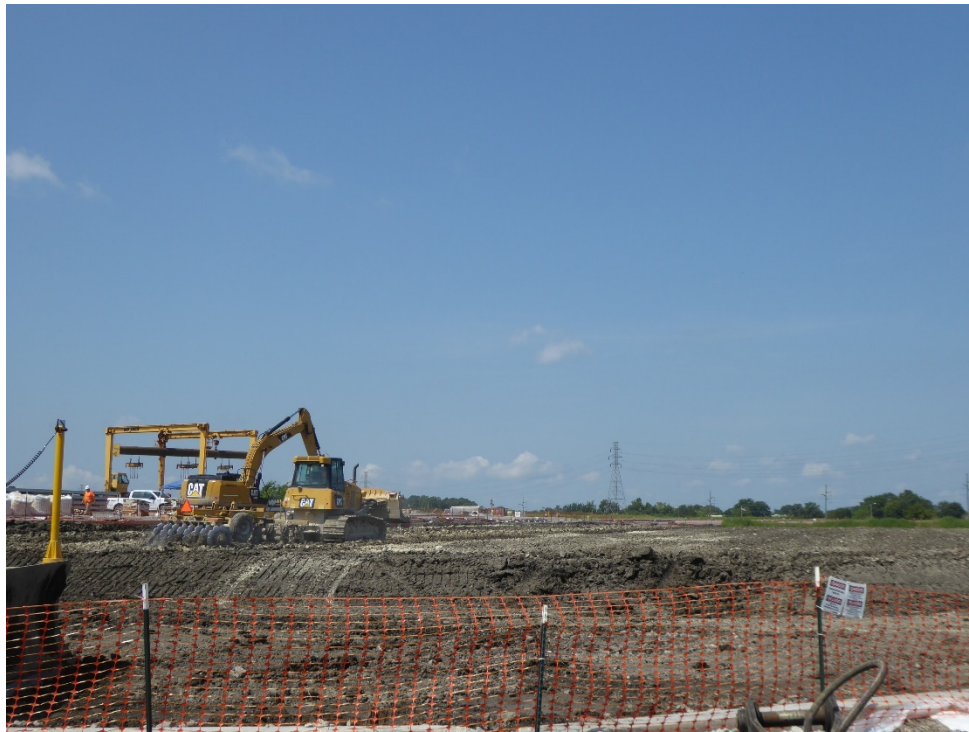
Application of amendment to dry out dredged sediment at southern part of CA2
