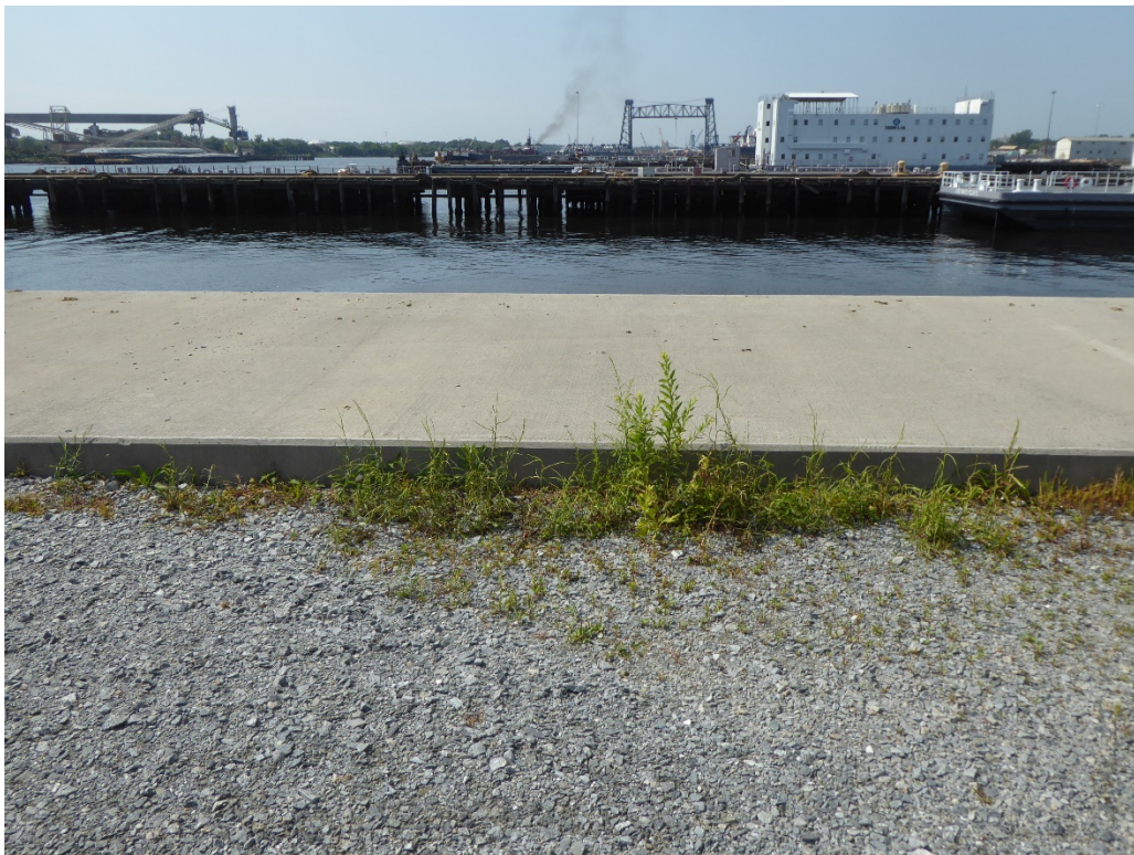
Evidence of CA1 settlement within offshore sheet pile containment wall
