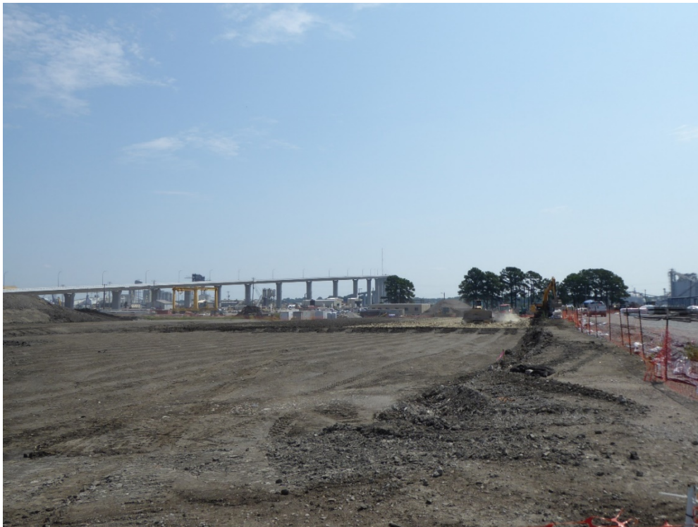
Grading of dredged material at CA2
