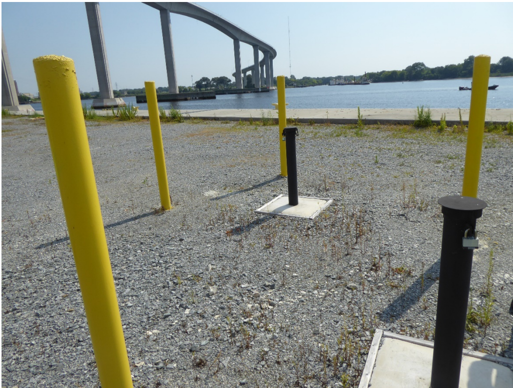
Locked monitoring wells in CA1
