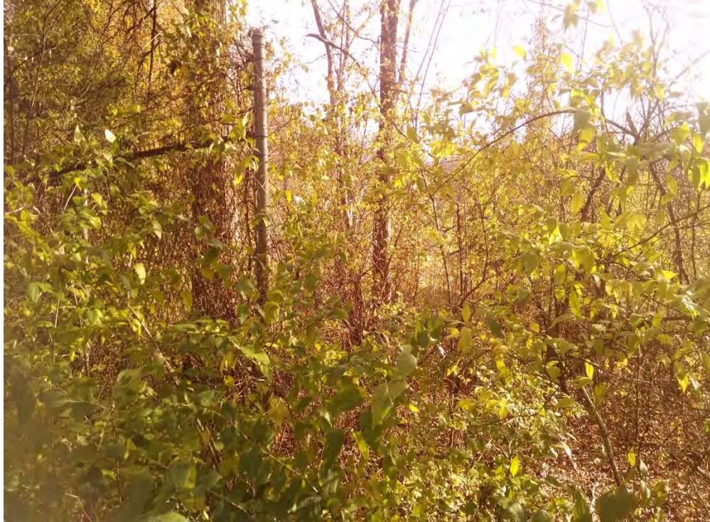
PHOTOGRAPH 01: Damaged fence on the northern edge of the Beaver Dam Road Land Fill
