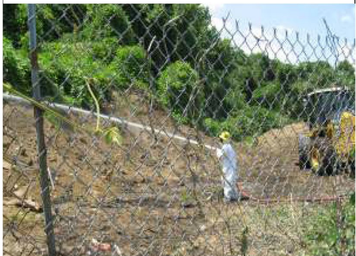
A certified EPA cleanup contractor sprays a portion of BoRit Asbestos Area site to suppress dust. This and many more safety measures are outlined in detail in the site's Health & Safety Plan, which you can view online.
