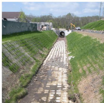
Top Left: Tannery Run before work began. Middle Left (2): Tannery Run was significantly widened to help reduce flooding. Geotextile and cabled concrete mats (CCMs), which are secured with specialized anchors that extend deep into the soil, line the open portion of the stream bed. Bottom Left: Gaps in the CCM were filled with soil and seeded. Top Right: Worker secures CCM. Bottom Right: By May 2011, plants had sprouted and held up well to heavy rains. Plants and their root systems play an important part in controlling erosion.
