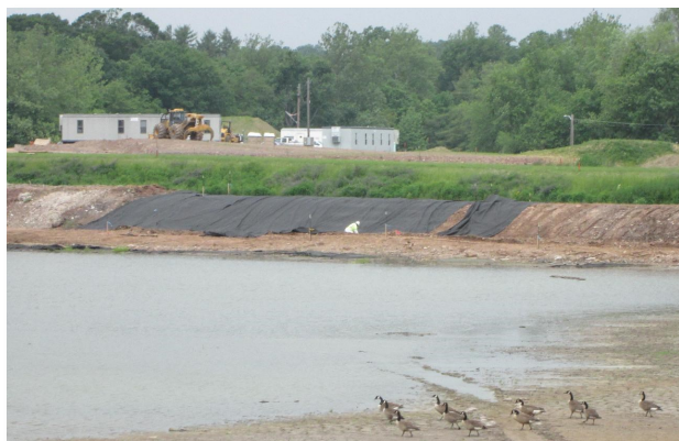
Geotextile fabric is laid on berm before clean material is placed.
