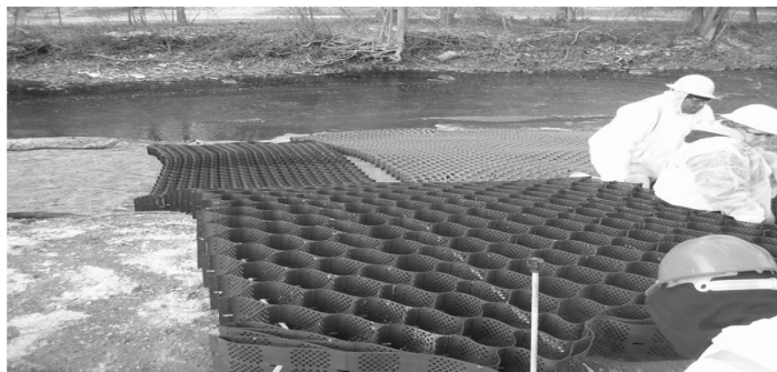
The photo above shows the geocells being used. Geocells are honeycomb-like structures made of plastic which can be filled with soil, stone, or concrete.
