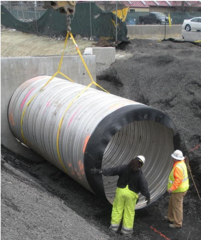
The 25-ft.-high embankment of Tannery Run, behind Butler Street businesses, was eroding and destabilizing parking lots. EPA enclosed a 325-foot portion of the stream to prevent collapse. Top Left: Crew installs the headwall to anchor the 8-ft-diameter pipe through which the stream will flow. Top Right: Water will flow from the lined open channel into the 8-ft. diameter pipe at the headwall. Bottom Left: Workers install first section of 8-ft-diameter pipe. Bottom Right: Liner and pipe were covered with 2,640 cubic yards of stone; the enclosed area was finished with soil and seeded.
