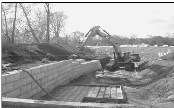
The photo above shows the retention wall being constructed (along the left) and the CCM placed on the stream bed.
