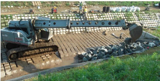
Top Left: Temporary pumps and a sand bag dam were installed to create a dry work area for rebuilding Rose Valley Creek. Upper Middle: Stream water was re-routed through 700 feet of piping and discharged into Wissahickon Creek while Rose Valley was being widened and lined. Lower Middle: Before geotextile and cabled concrete mats (CCM) were laid, workers placed a layer of stone on the floor of Rose Valley Creek. Bottom Left: For added security, rip rap was placed over the CCM on the stream embankment. Top Right: Rose Valley Creek after being repaired and widened to reduce future flooding.
