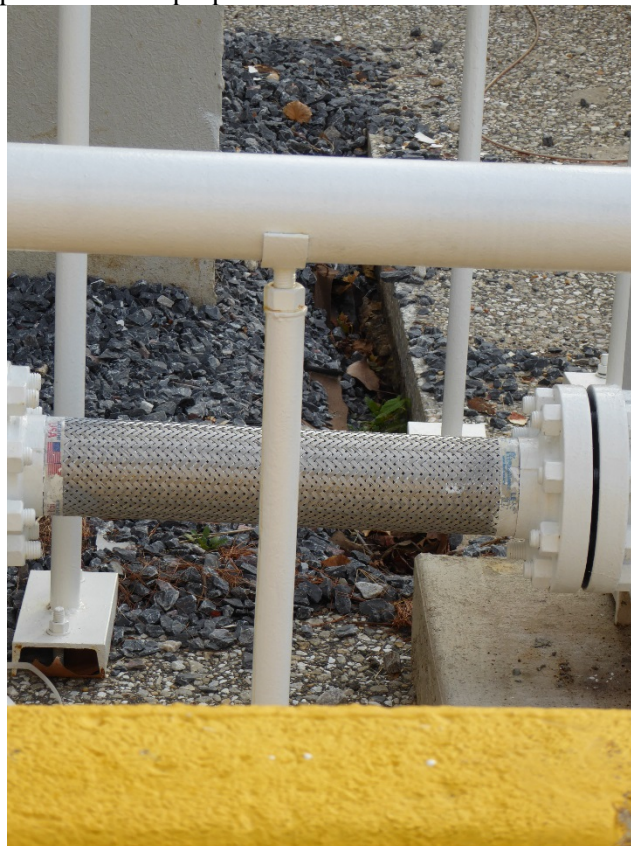
Area where asphalt cap was cut and removed during propane tank installation at the Treatment Yard area
