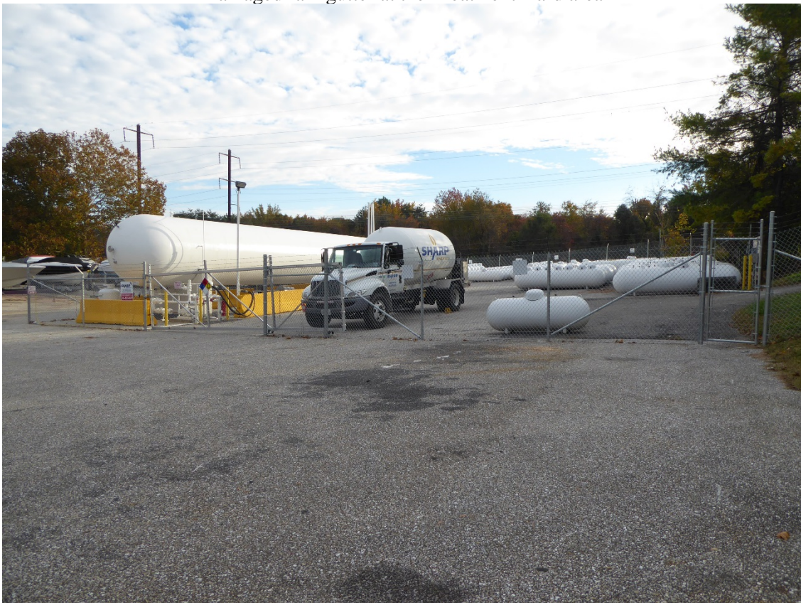
Propane distribution business on the Treatment Yard area
