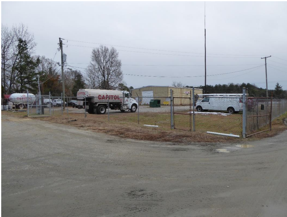
Looking south on parcel 7986773046 and the Capitol Oil office building
